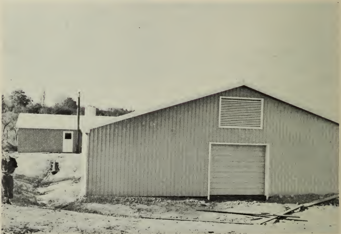
Figure 9. A windowless laying house showing a louver that lets air into the attic.
