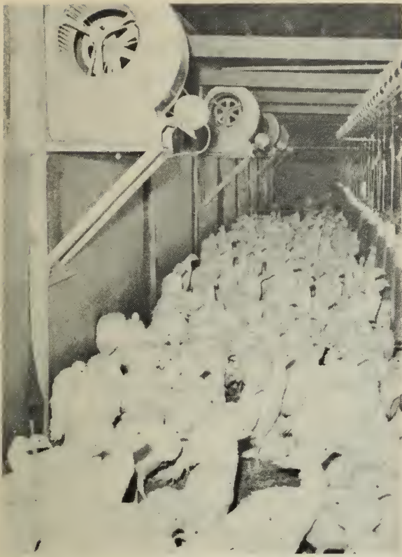
Figure 7. Centrifugal fans ventilating a turkey broiler pen.
