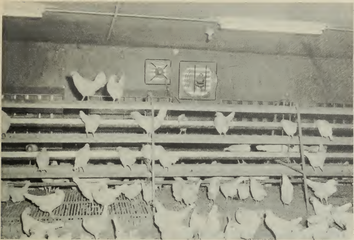
Figure 24. A laying house ventilated by a continuously operating small fan and a larger fan controlled by a thermostat. Note the feed and water over the dropping pits.
