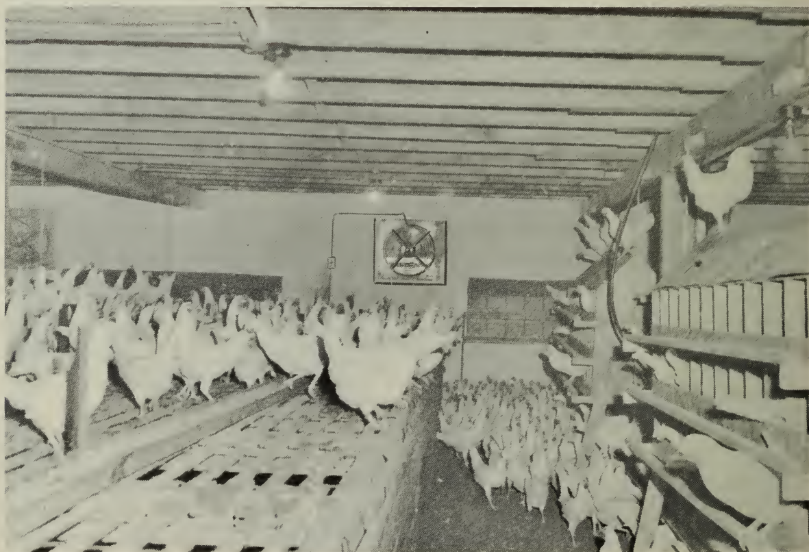
Figure 5. A small-diameter propeller fan ventilating a laying house.
