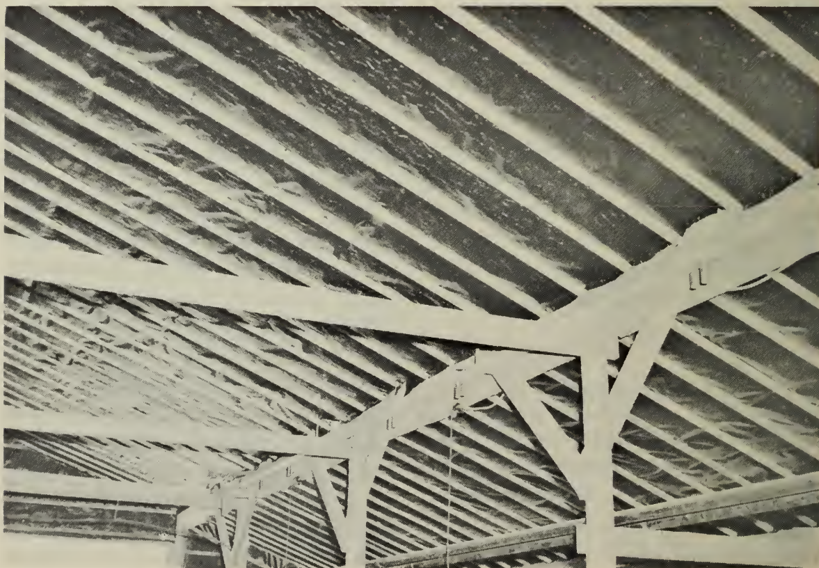
Figure 2. A broiler house in which insulation was added to the roof to permit better ventilation.
