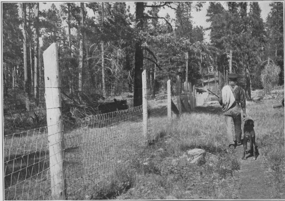
A COYOTE-PROOF PASTURE FENCE IN THE IMNAHA NATIONAL FOREST, OREGON, CONSTRUCTED TO TEST THE FEASIBILITY AND ECONOMY OF GRAZING SHEEP WITHOUT A HERDER.
