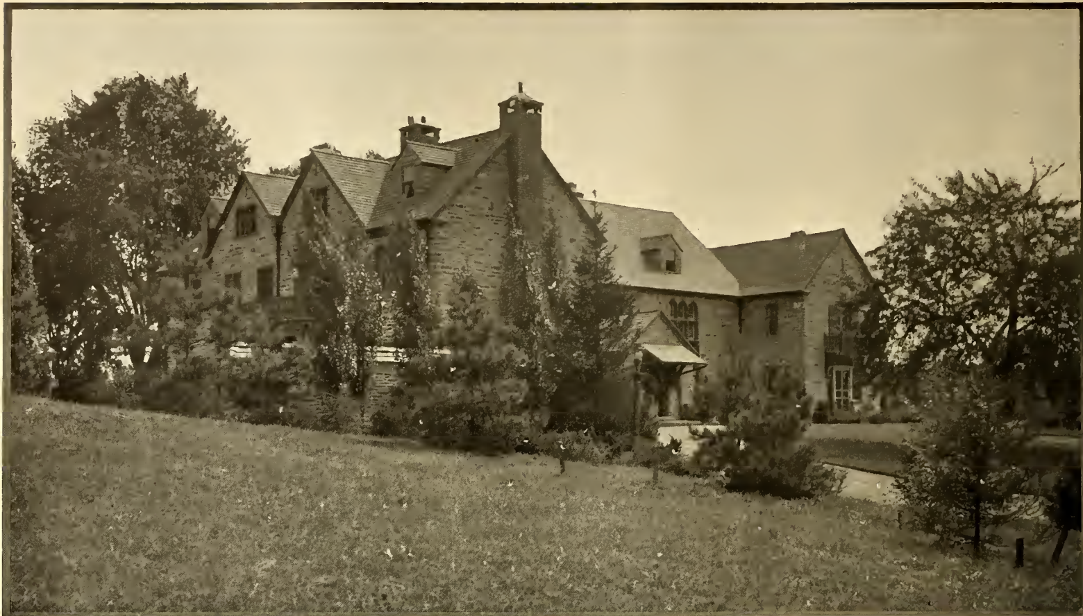
The north front of Fox Hill Farmhouse at Radnor, Pennsylvania
