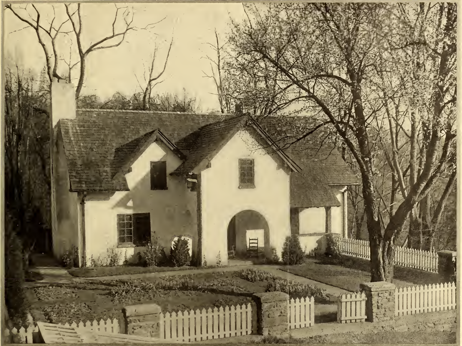
The garden front of Krisheim Cottage, a small house of distinction at St. Martins, Pennsylvania
