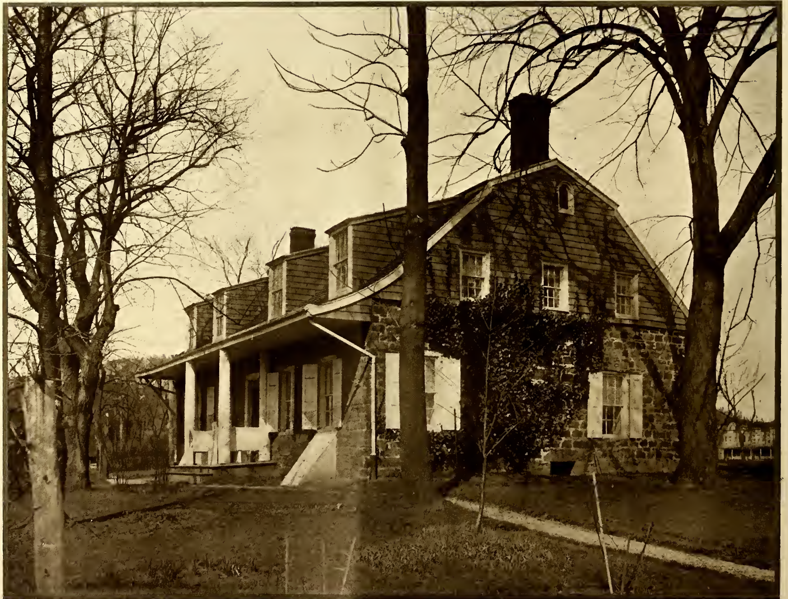
The eastern end of the house, showing the width of the eaves and the unusual arrangement of columns about the doorway
