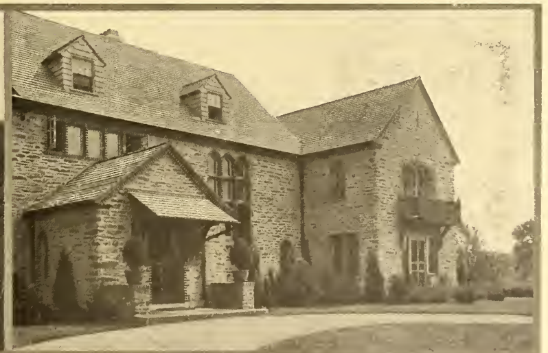
The low, hooded porch on the north front
