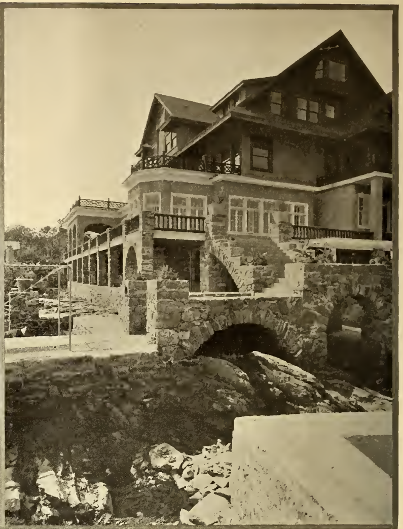
Steps leading to the terrace
