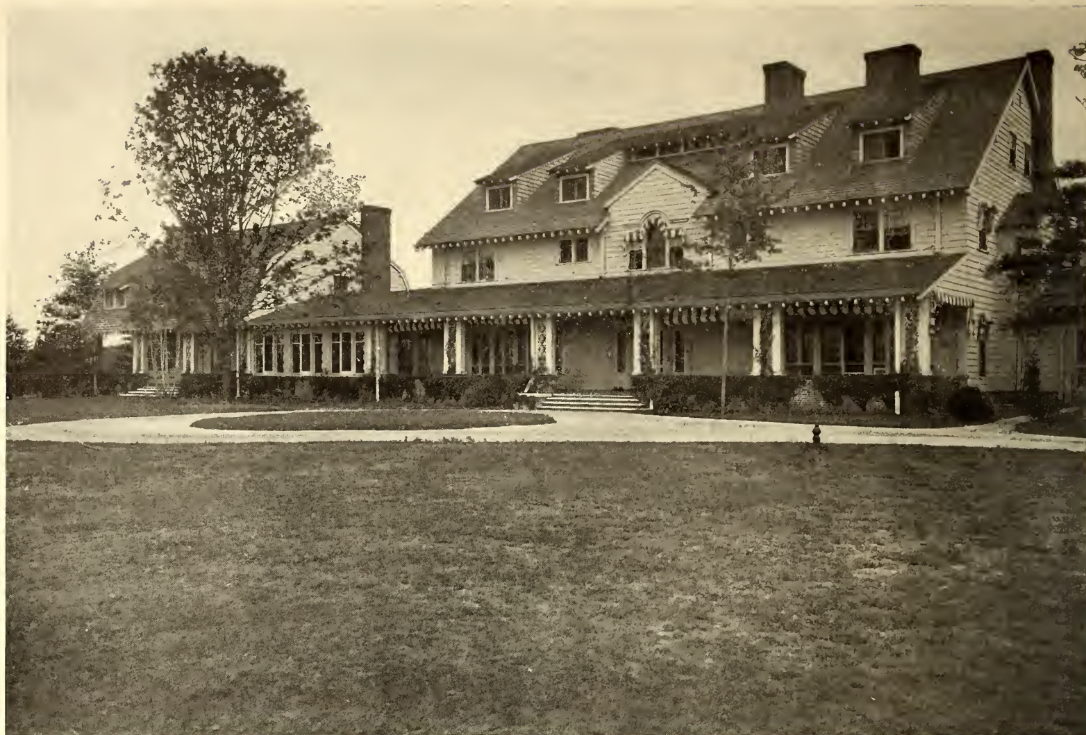
This delightfully commodious country home near Manhasset, Long Island, consists of what is practically a group of connected buildings
