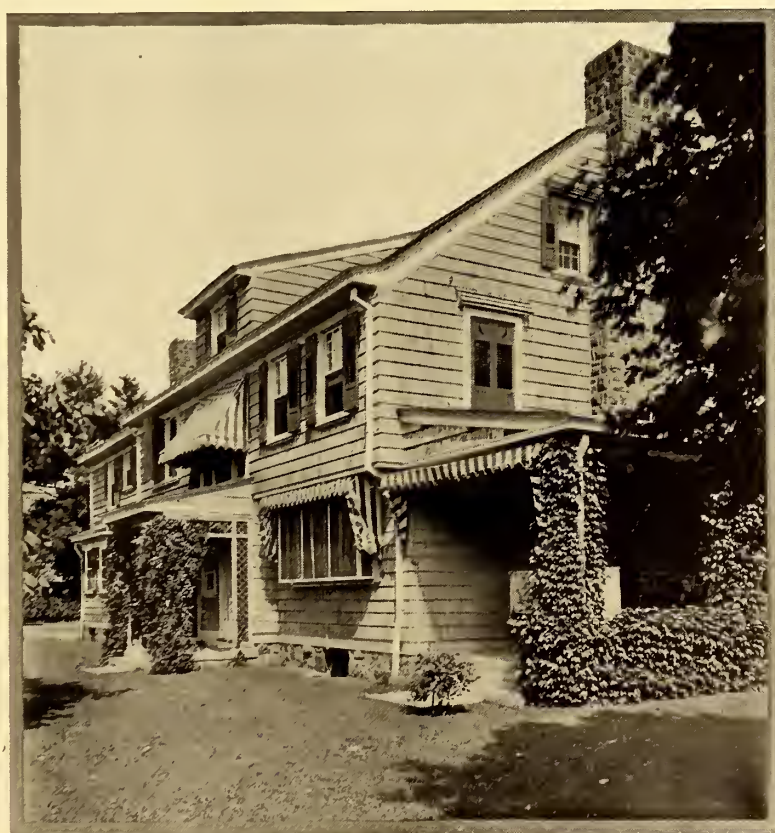
The veranda end of the house
