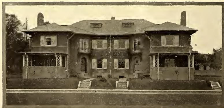
This is an excellent example of a double house. The entrance doors and wrought iron balconies are worthy of note. The first and second story plans of the right hand half of this are here shown
