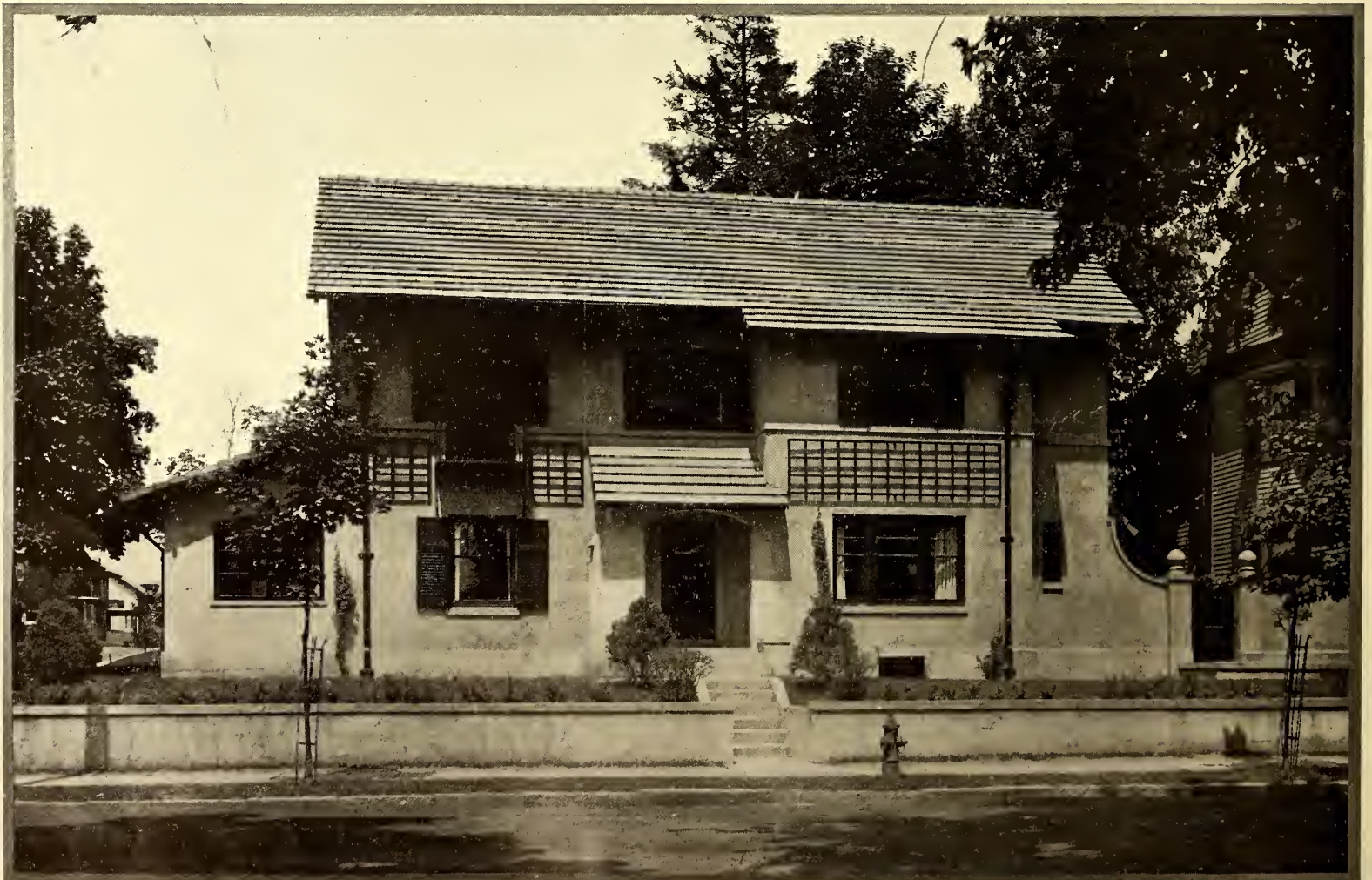
The lattice and the leaders add to the decorative quality of this exterior. The wall and gate screening the service yard from the street is an interesting conception
