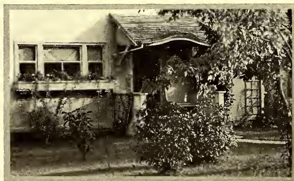
Entrance Porch, Campbell house
