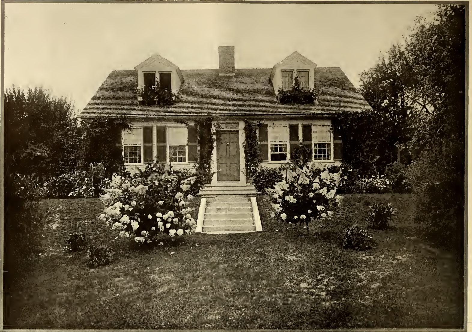
This delightful cottage is one of the most successful recent experiments in remodeled farmhouses
