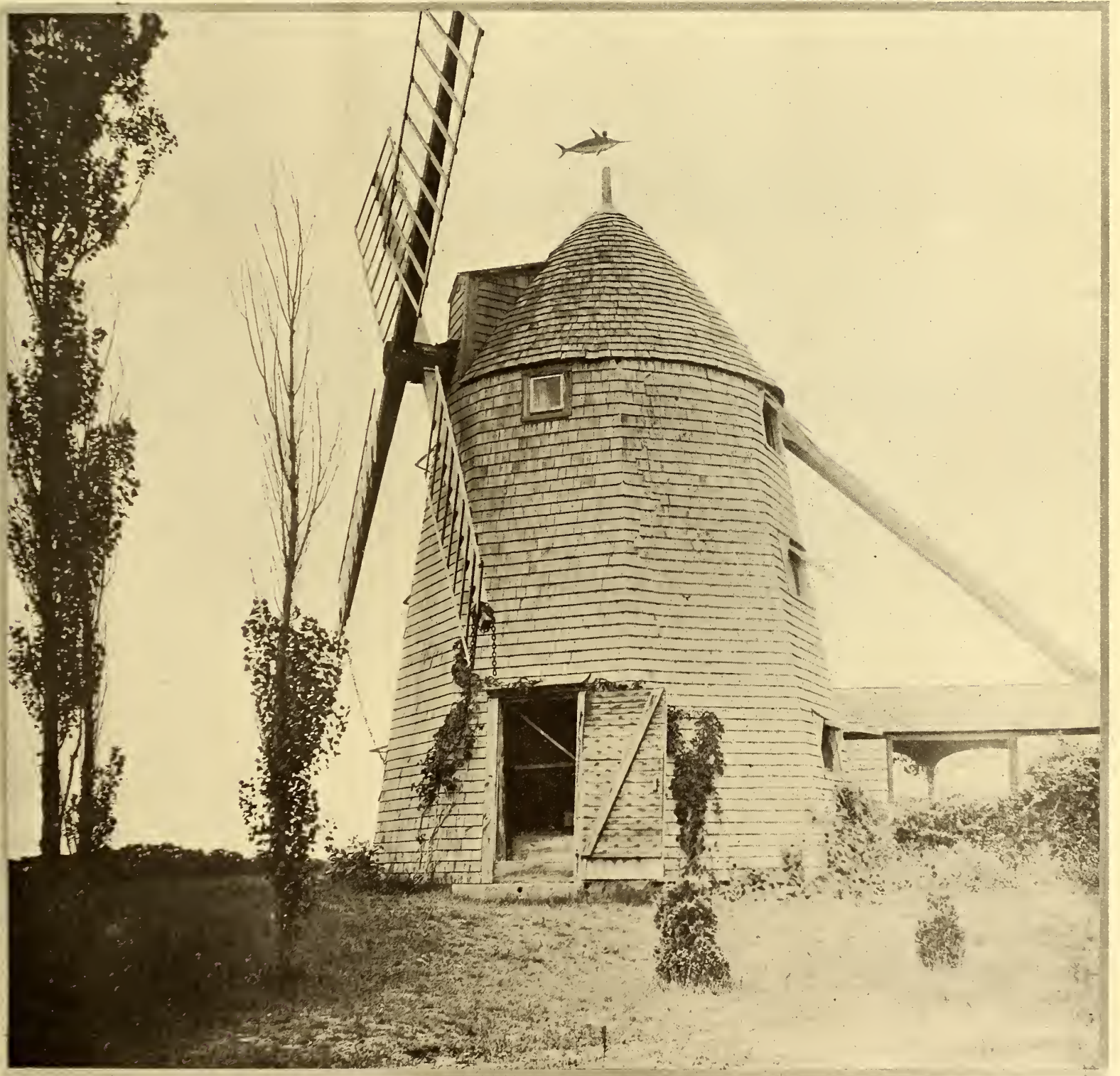
Original entrance door to the old mill
