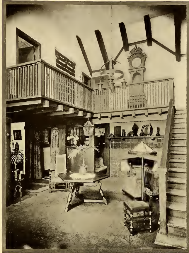
Balcony in the living-room
