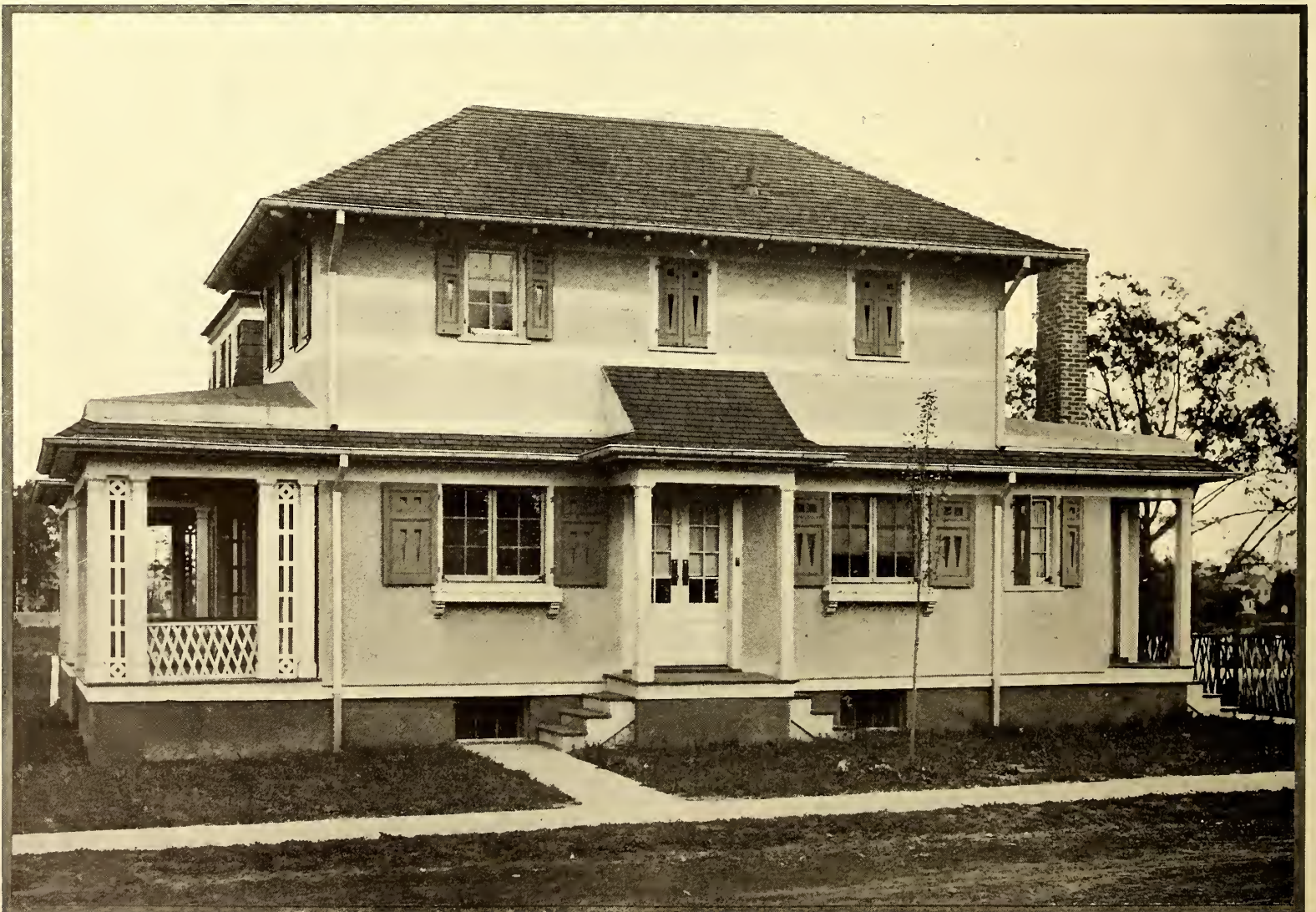
A stucco house at Cedar Manor, Jamaica, Long Island, New York
