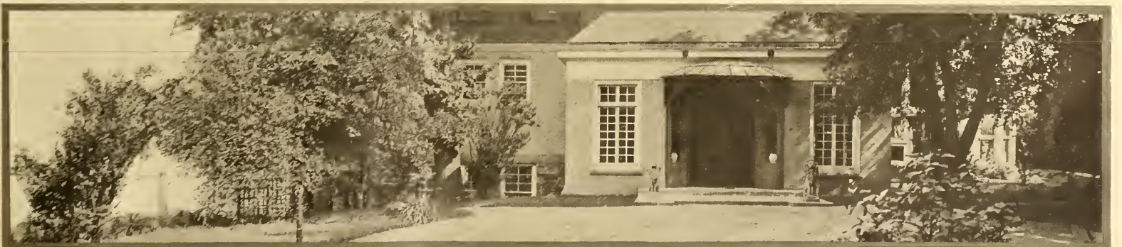
The lawn front of the house, with its broad entrance doorway, faces a situation in charming contrast with the water view
