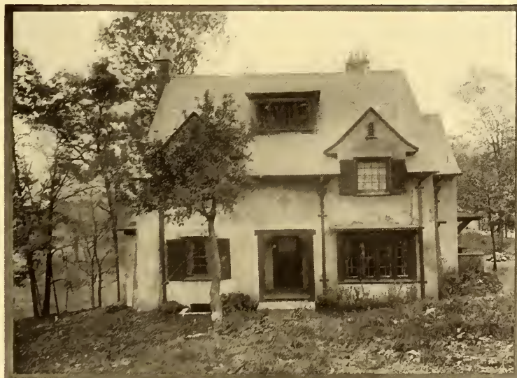
Entrance front of the Bacon House
