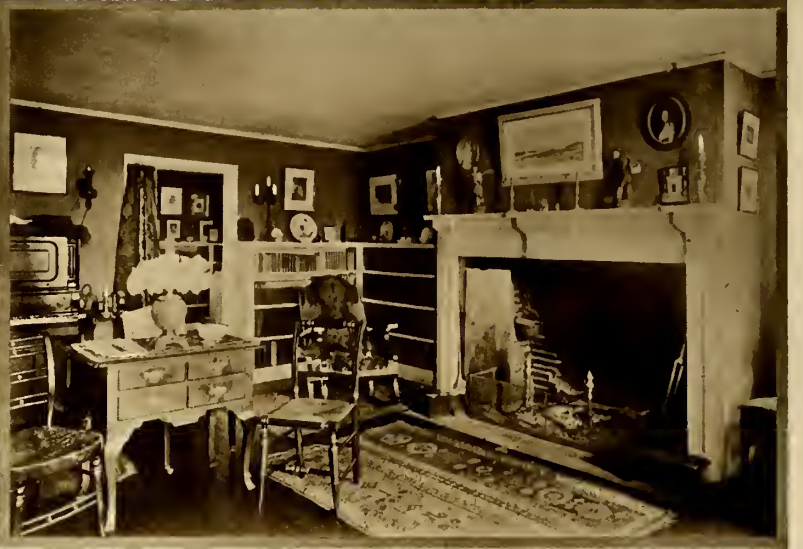
The great fireplace with its original crane and pot
