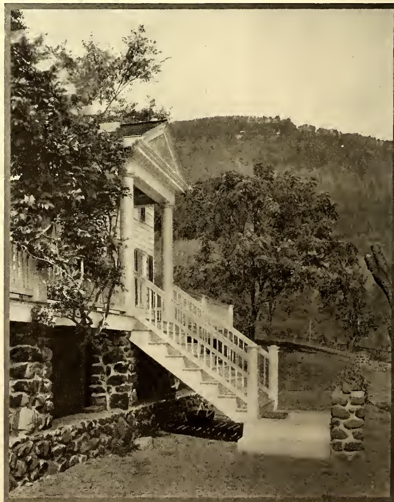
Steps to the entrance-porch
