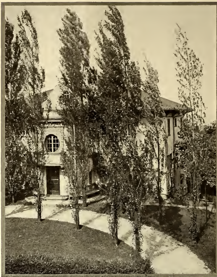
Entrance doorway of Mr. E. Spencer Hall's house
