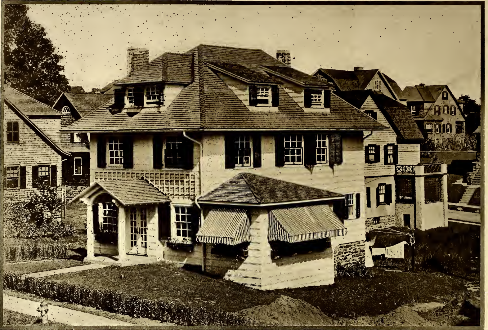
The small site on sloping ground has been well employed in the type of house chosen to fit it, as shown above
