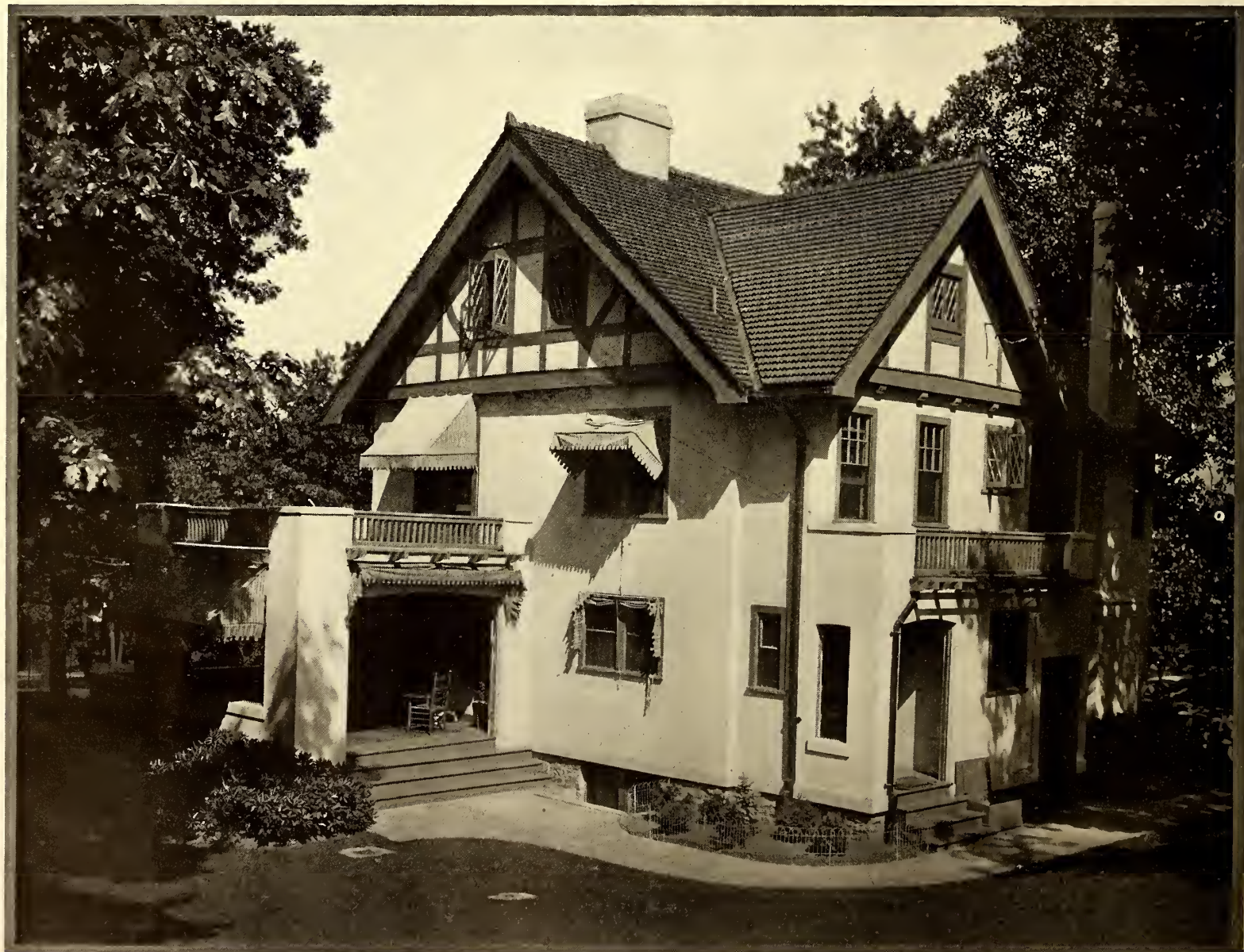
Garden side of the Master house
