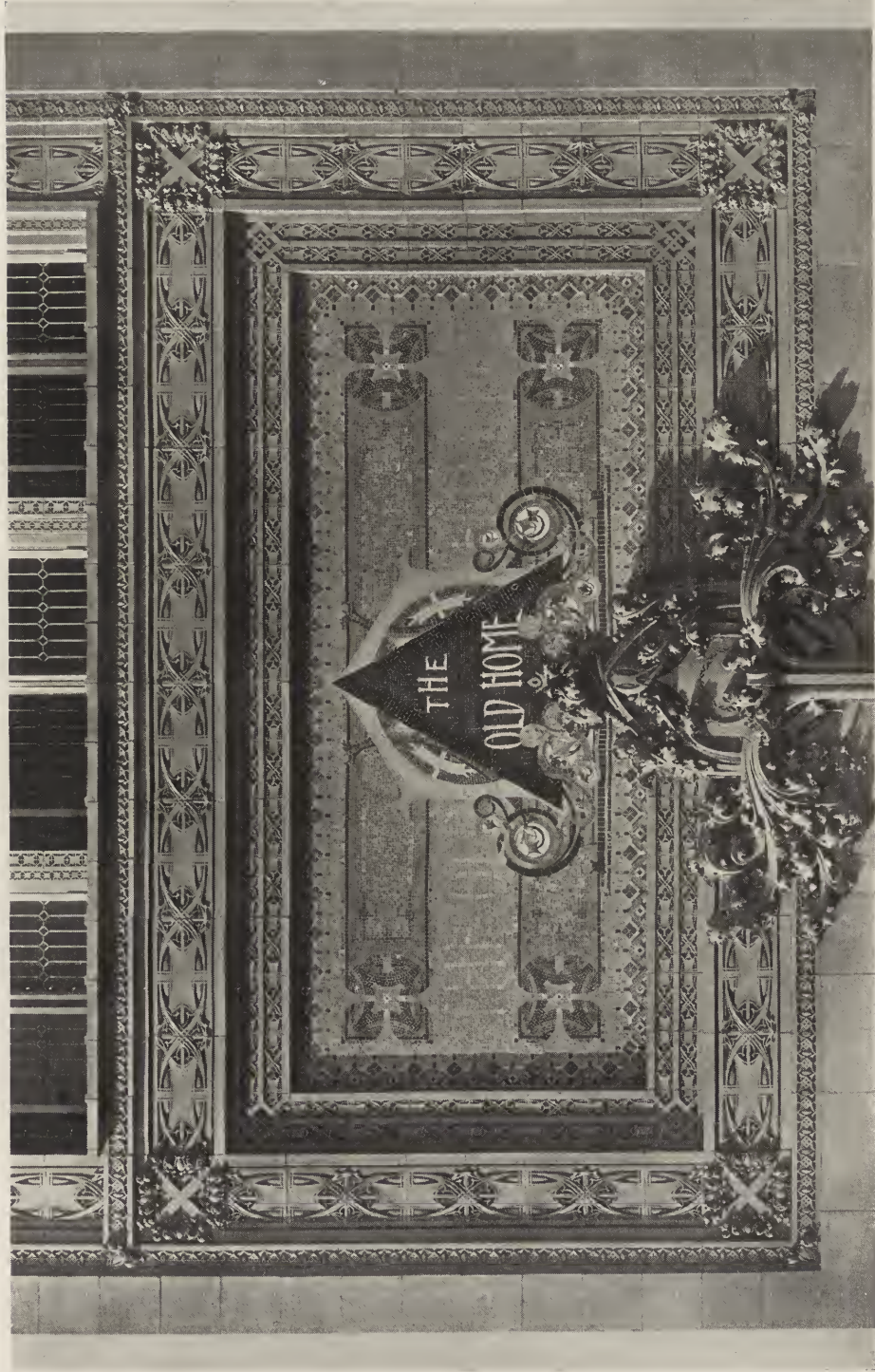
DETAIL OF POLYCHROME GLASS MOSAIC PANEL, EAST FRONT—THE HOME BUILDING ASSOCIATION COMPANY, NEWARK, OHIO. LOUIS H. SULLIVAN, ARCHITECT.
