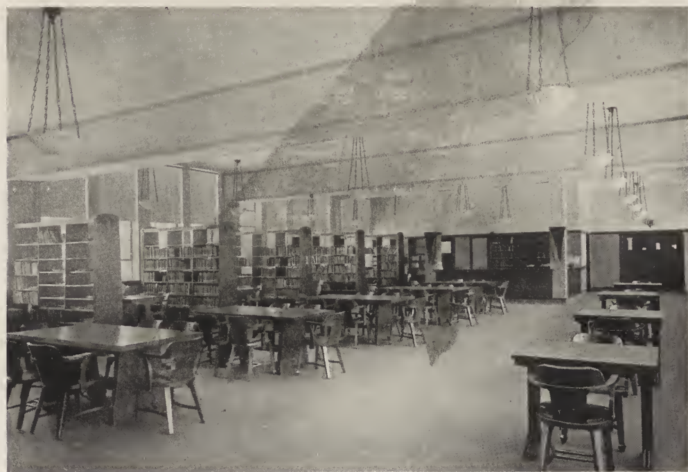
FIG. 16. LIBRARY ON THIRD FLOOR OF WEST BUILDING, SHOWING PLAIN REINFORCED BEAMS WITHOUT DECORATIVE MOULDINGS, SPAN THIRTY-EIGHT FEET—Y. M. C. A. COLLEGE, CHICAGO.
