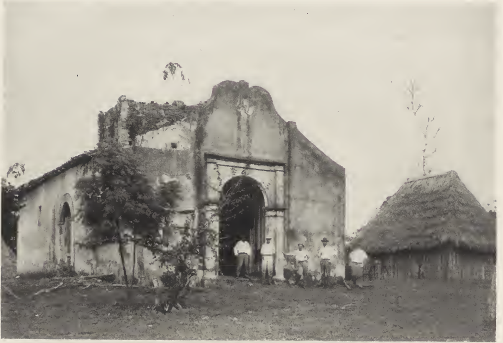
CHURCH AND SCHOOL HOUSE, ARRAJAN, PANAMA.
