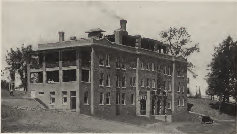
FIGS. 52, 53 AND 54. FLOOR PLANS AND VIEW OF EXTERIOR—BARRE (VERMONT) CITY HOSPITAL. EDWARD F. STEVENS, ARCHITECT.
