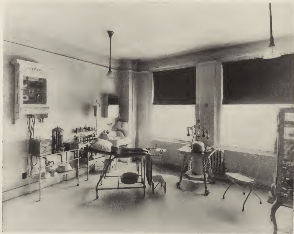
VIEW OF OPERATING ROOM—COBB BUILDING, SEATTLE, WASH. Howells & Stokes, Architects.
