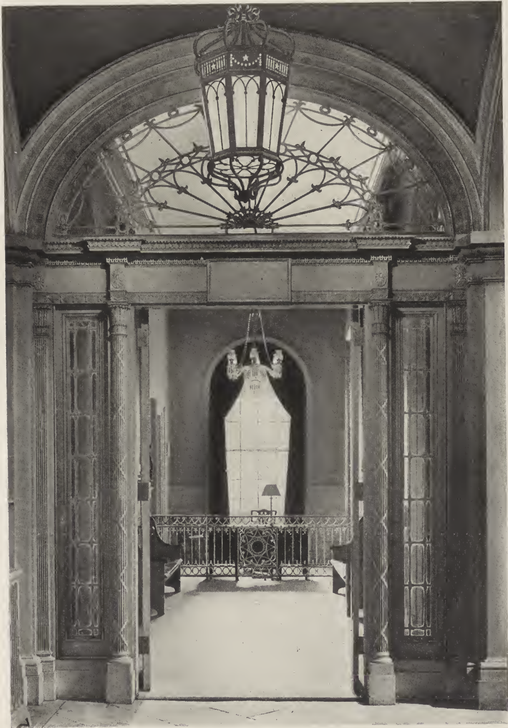
SCREEN AT EAST END OF MAIN CORRIDOR—NEW YORK CITY HALL. GROSVENOR ATTERBURY, ARCHITECT FOR THE RESTORATION. JOHN TOMPKINS AND STOWE PHELPS, ASSOCIATED.
