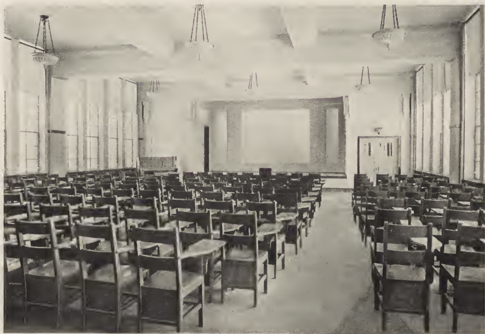
FIG. 15. CHAPEL AND SECTION ROOM ON SECOND FLOOR OF WEST SECTION, SHOWING REINFORCED CONCRETE GIRDERS IN CEILING WITH SPAN OF THIRTY-EIGHT FEET—Y. M. C. A. COLLEGE, CHICAGO.
