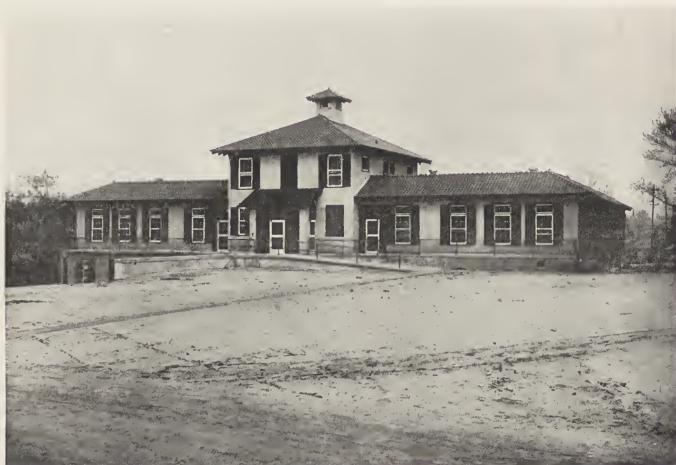
FIG. 48. VIEW OF WHITE ISOLATION BUILDING, ST. LUKE'S HOSPITAL, JACKSONVILLE, FLA. Edward F. Stevens, Architect; Mellen C. Greeley, Associate Architect.
