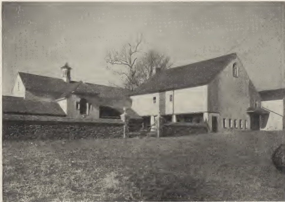
BARN AND POLO STABLES FOR A. J. DREXEL PAUL, ESQ., RADNOR, PA. Mellor & Meigs, Architects.
