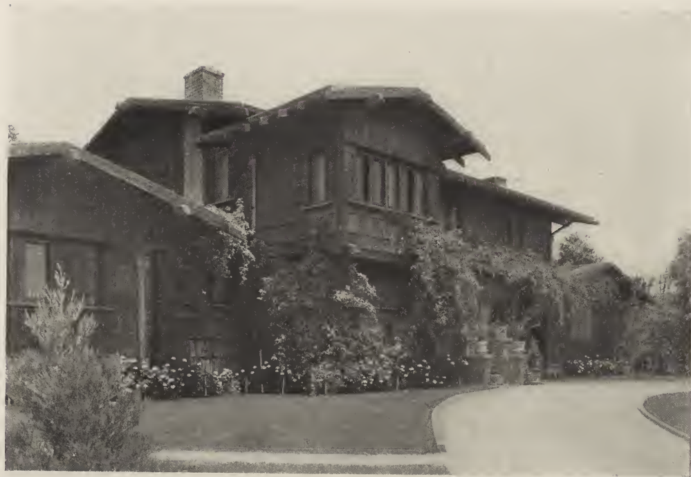
RESIDENCE OF WILLIAM A. CHILDS, ESQ., RIVERSIDE, CAL. George A. Clark, Architect.
