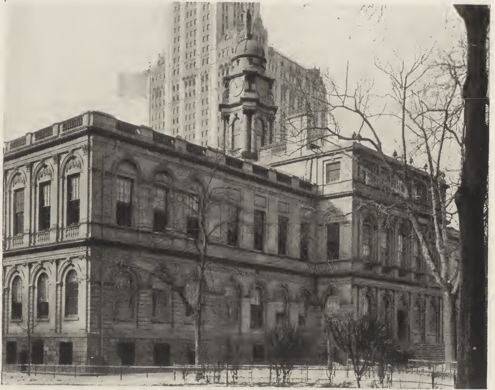
THE NEW YORK CITY HALL, FROM THE NORTHEAST. THE BROWNSTONE WALLS ON THE REAR ARE PAINTED TO THE TONE OF THE ADJOINING MARBLE.
