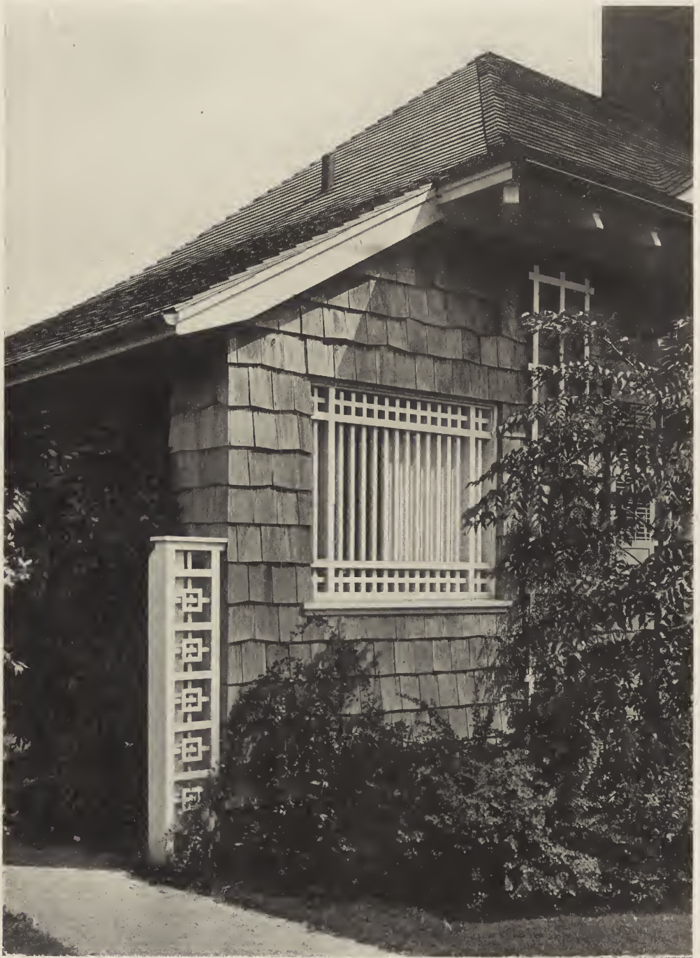
DETAIL OF SERVICE WING—COUNTRY HOUSE AT SOUTHAMPTON, L. I. GOODHUE LIVINGSTON, ESQ., OWNER AND ARCHITECT.
