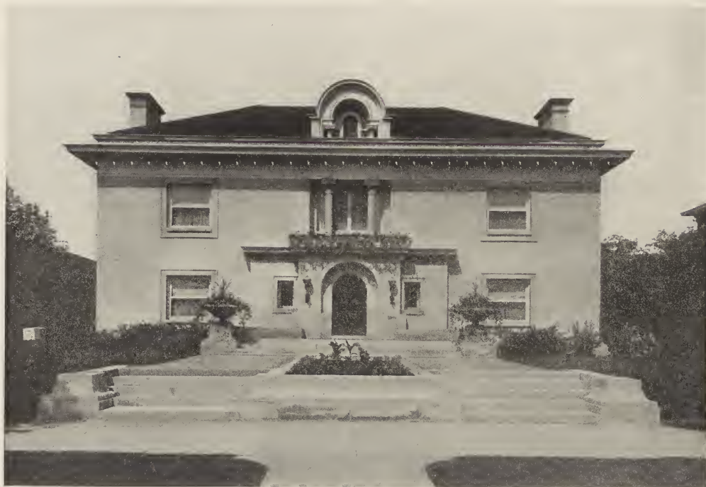
RESIDENCE OF EDWIN M. COLVIN, ESQ., CHICAGO. George W. Maher, Architect.
