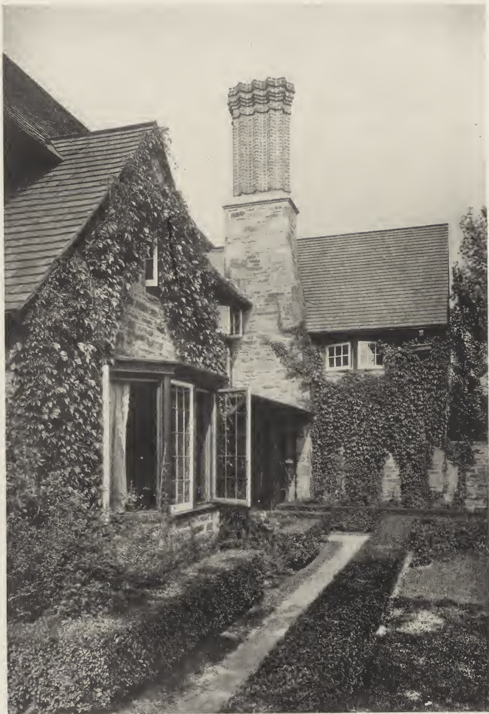
LIVING ROOM BAY—HOUSE AT CYNWYD, PA. MELLOR & MEIGS, ARCHITECTS.
