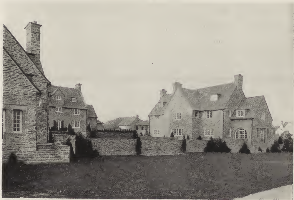
FROM LOWER OR SUNKEN GARDEN—GROUP OF THREE RELATED HOUSES ON WILLOW GROVE AVENUE. Robert Rodes McGoodwin, Architect.
