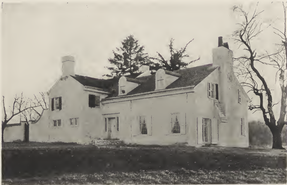
REAR VIEW—PICKERING HUNT CLUB, PHOENIXVILLE, PA. Mellor & Meigs, Architects.
