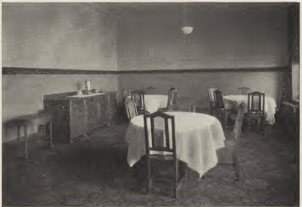
SECOND OFFICERS' DINING ROOM—PENN MUTUAL BUILDING, PHILADELPHIA. Edgar V. Seeler, Architect.
