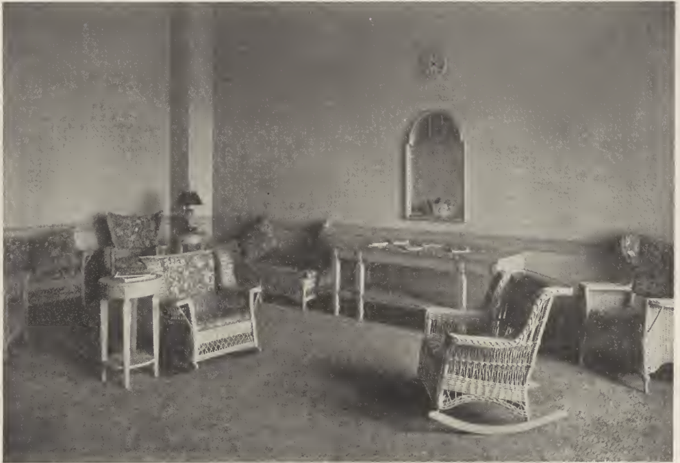
WOMEN'S REST ROOM—PENN MUTUAL BUILDING, PHILADELPHIA. Edgar V. Seeler, Architect.
