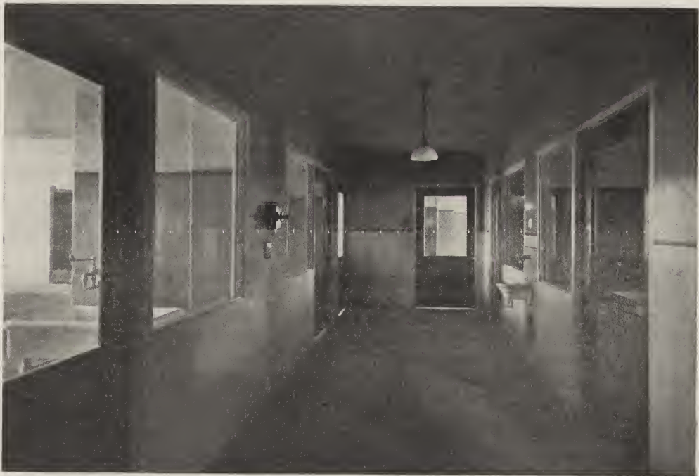
FIG. 30. ISOLATION DEPARTMENT CORRIDOR—OHIO VALLEY GENERAL HOSPITAL, WHEELING, W. VA.
