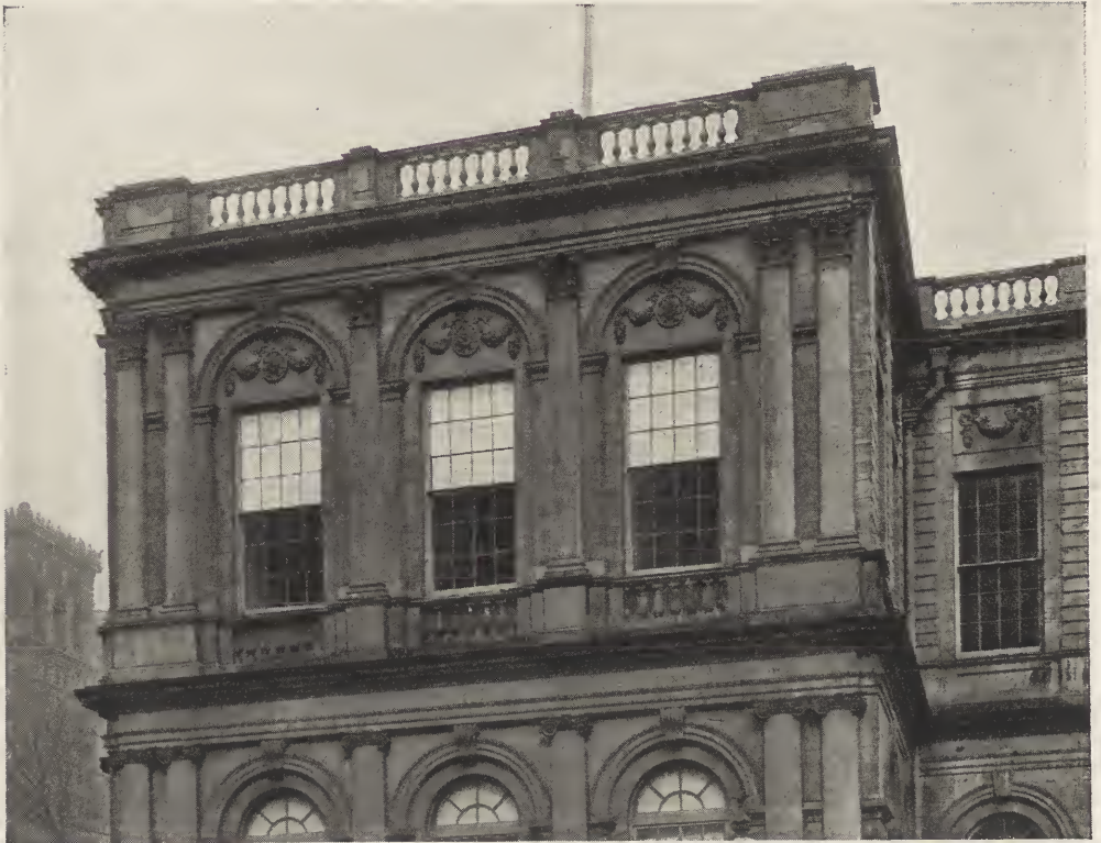
DETAIL AT SECOND FLOOR, SOUTH FRONT.
