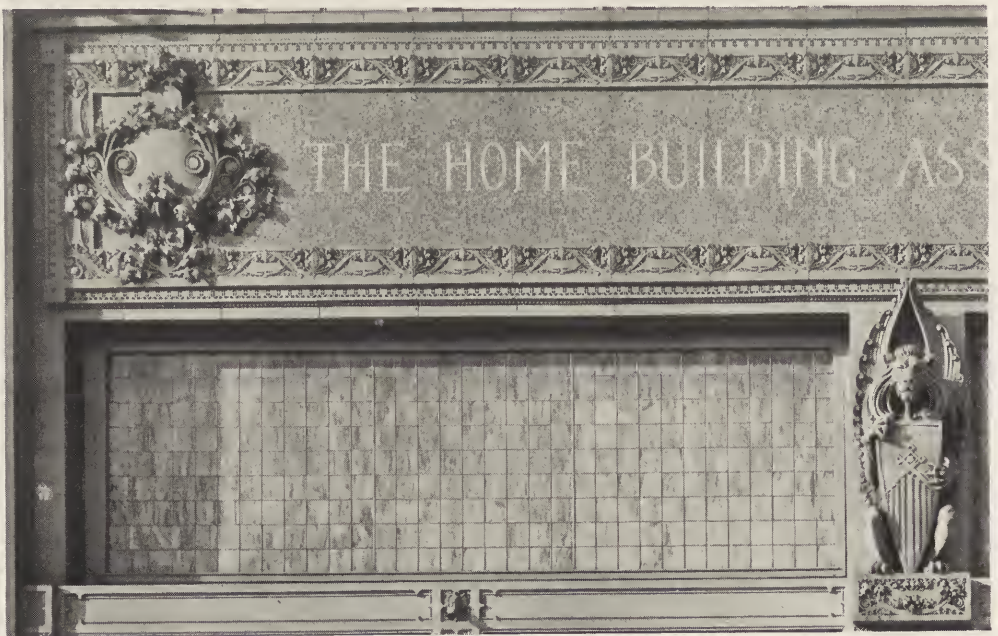
DETAIL OF GLASS MOSAIC PANEL, SOUTH FRONT—THE HOME BUILDING ASSOCIATION COMPANY, NEWARK, OHIO. Louis H. Sullivan, Architect.
