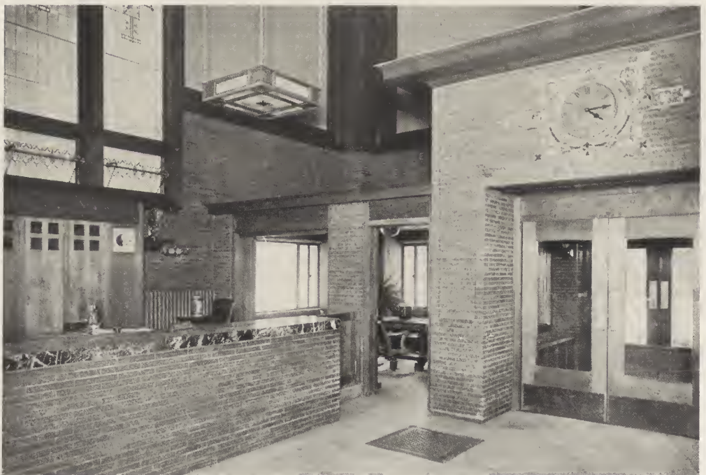
INTERIOR VIEW, SHOWING OFFICERS' QUARTERS AND PRESIDENT'S ROOM. Louis H. Sullivan, Architect.
