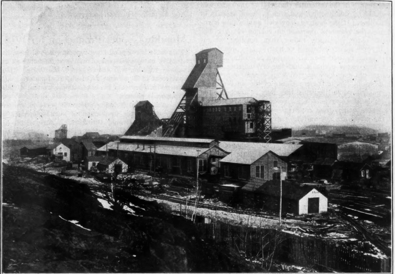
SHAFTS AT THE CREIGHTON MINE (NICKEL-COPPER) OF THE CANADIAN COPPER CO., AT CREIGHTON, ONTARIO
