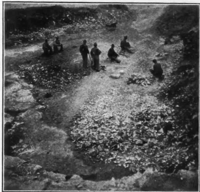
HAND QUARRYING PENDING ARRIVAL OF CRUSHER
