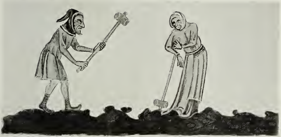
BREAKING CLODS OF EARTH WITH MALLETS
