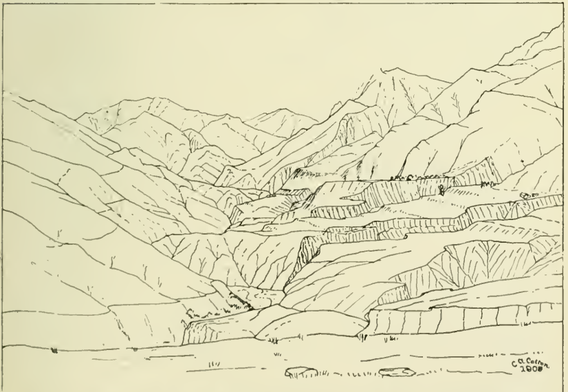
FIG. 237.—View of terraces in the Shotover Valley, N.Z., looking southward down the valley. The alluvium forming the terraces is partly sluiced away. The river-banks are solid schist rock.
