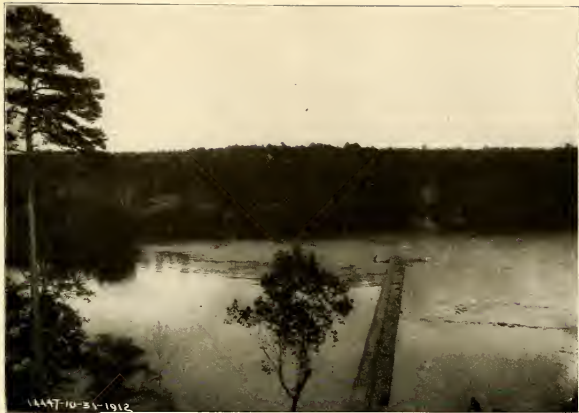
COOSA RIVER, LOCK 12 DAM IN PROCESS OF CONSTRUCTION
