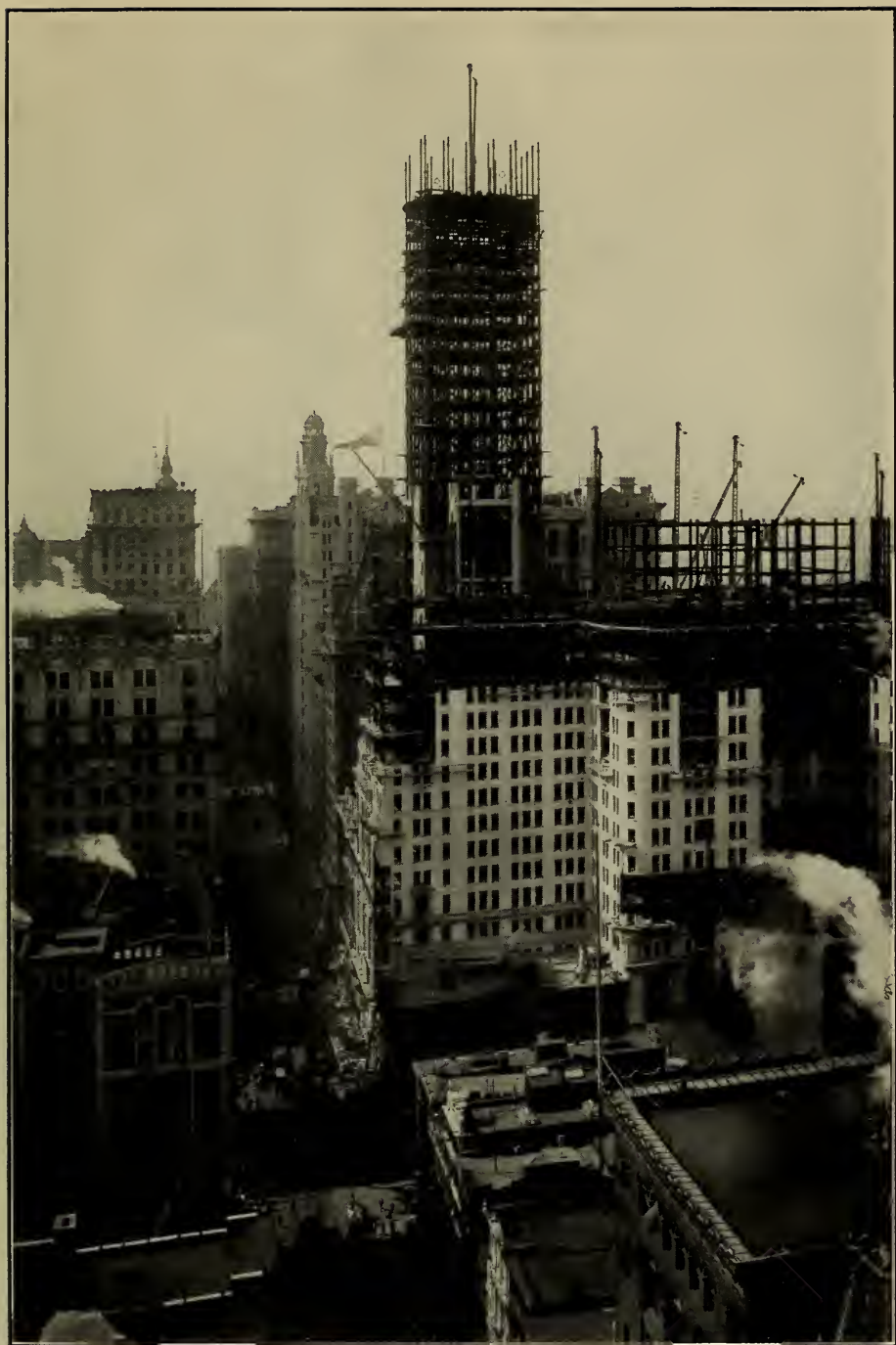
SKYSCRAPERS IN PROCESS OF CONSTRUCTION.
