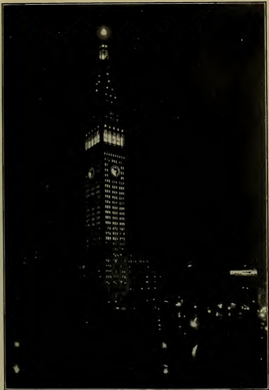
THE TOWER OF THE METROPOLITAN-LIFE BUILDING, NEW YORK, ILLUMINATED.
