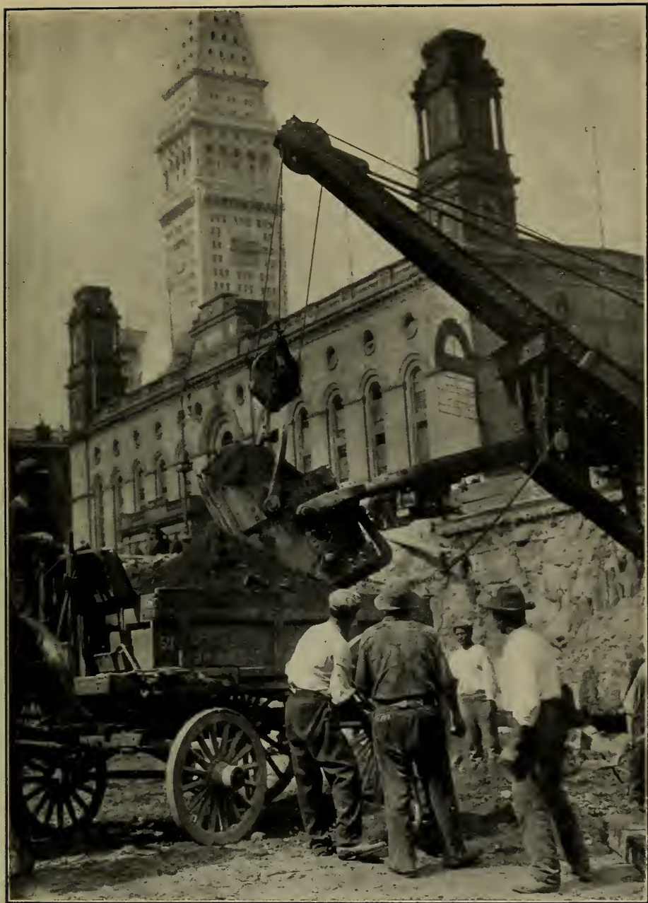
EXCAVATING FOR THE FOUNDATION OF A SKYSCRAPER.
