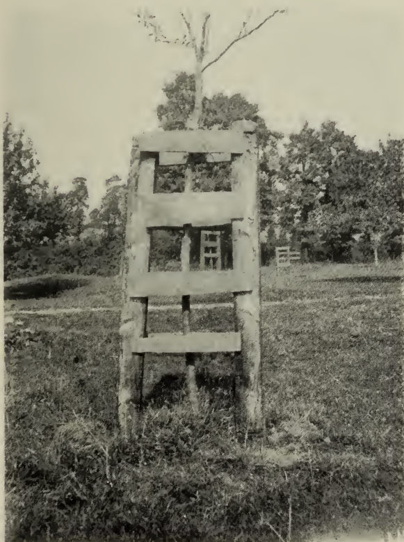
FIG. 138.—FENCING WITH OLD RAILWAY SLEEPERS AND BARREL STAVES.
