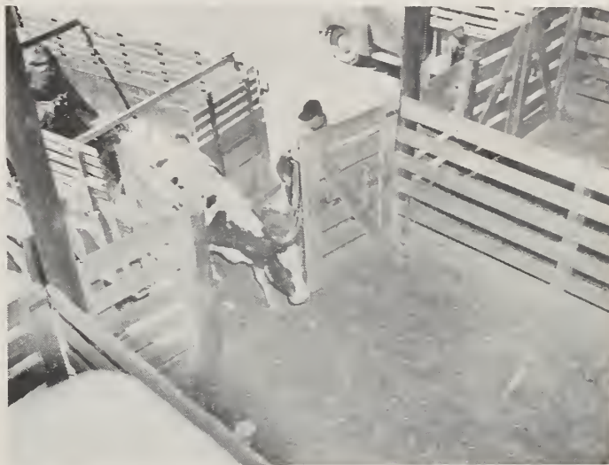
N-24738--Individual consignments are kept in separate enclosures having gates that swing both ways to form pens and alleys. Platform of unloading dock is same height as floor of truck to facilitate unloading.
