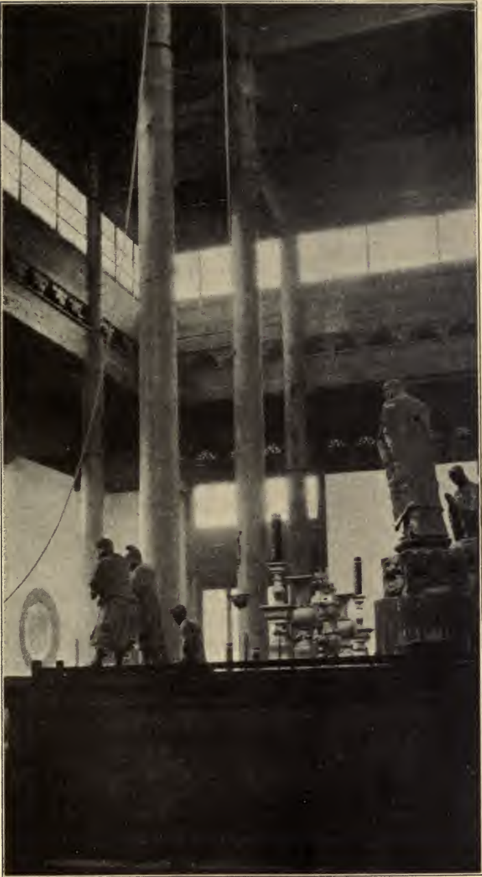
AMERICAN SPARS USED IN THE RECONSTRUCTION OF LING YING TEMPLE
