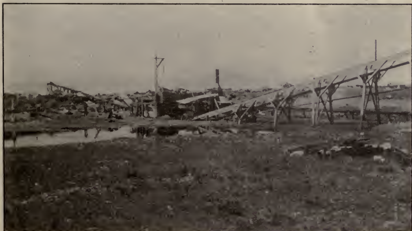
Oro Del Norte Black Sands Plant, showing method of hauling sands to bins on incline trestle.
