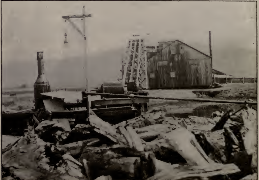
Oro Del Norte Black Sands Plant, showing the revolving screen.
