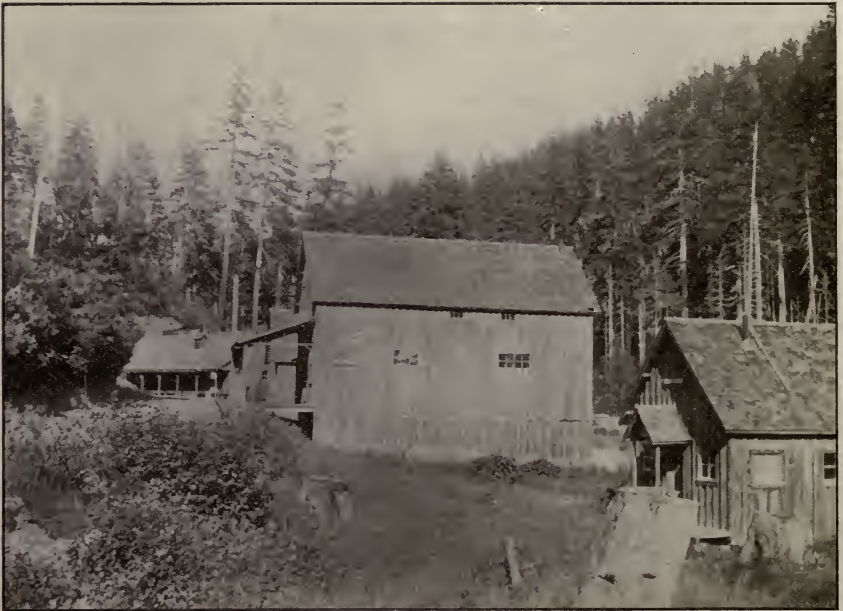
Monumental Mine buildings at Monumental, Del Norte County, California.
