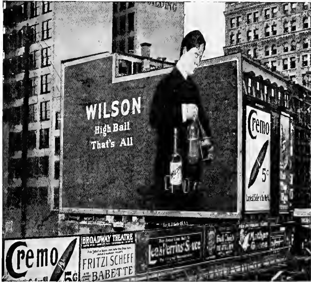
A PAINTED WALL WITH HEAD OF THE MAN BUILT UP AND CUT OUT.
