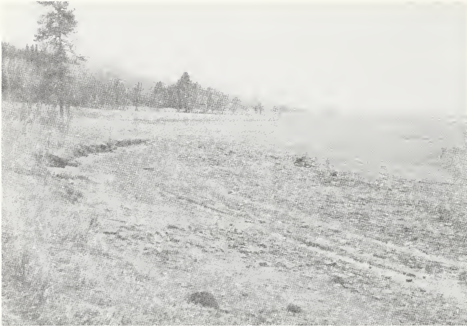
Fig. 10. Looking north at 10-VY-336 showing the depth of erosion caused by the reservoir.
