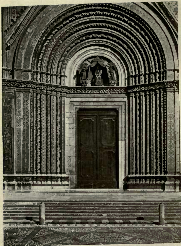
Porta centrale. Central door.
