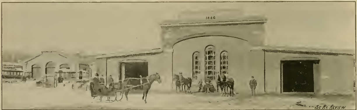
STABLES, WITH REPAIR SHOP TO THE LEFT—MONTREAL STREET RAILWAY.
