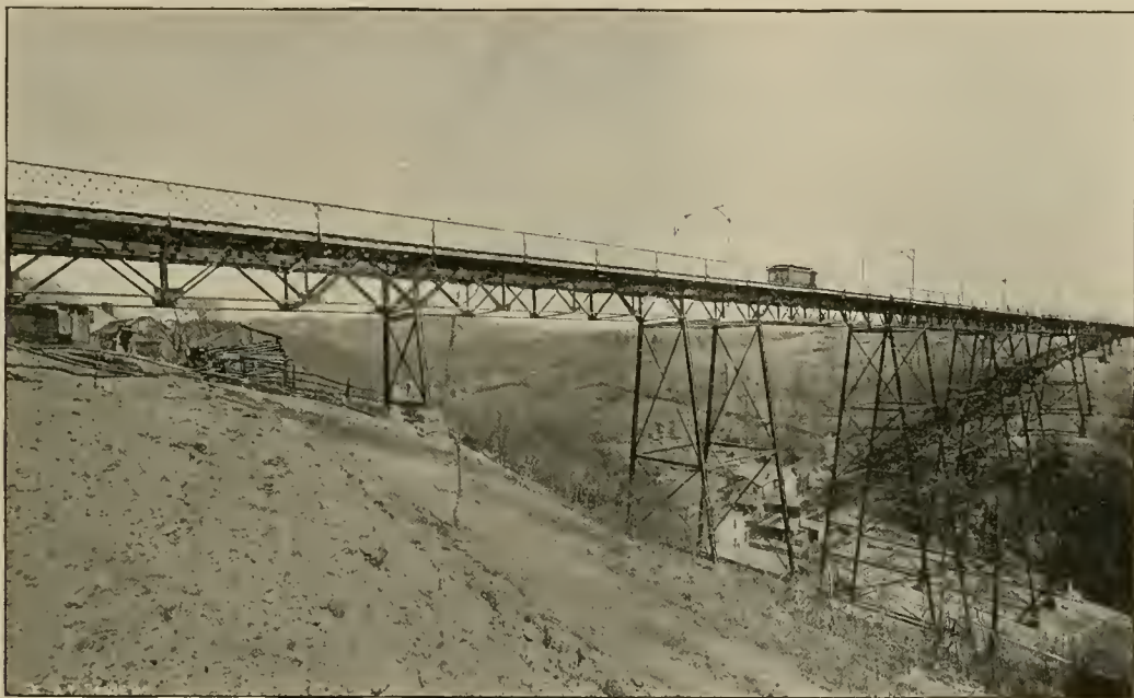
OVER JACK'S RUN, 167 FEET ABOVE THE VALLEY.
