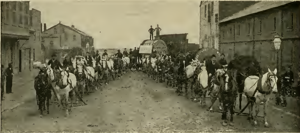
FORTY TONS OF CABLE.
