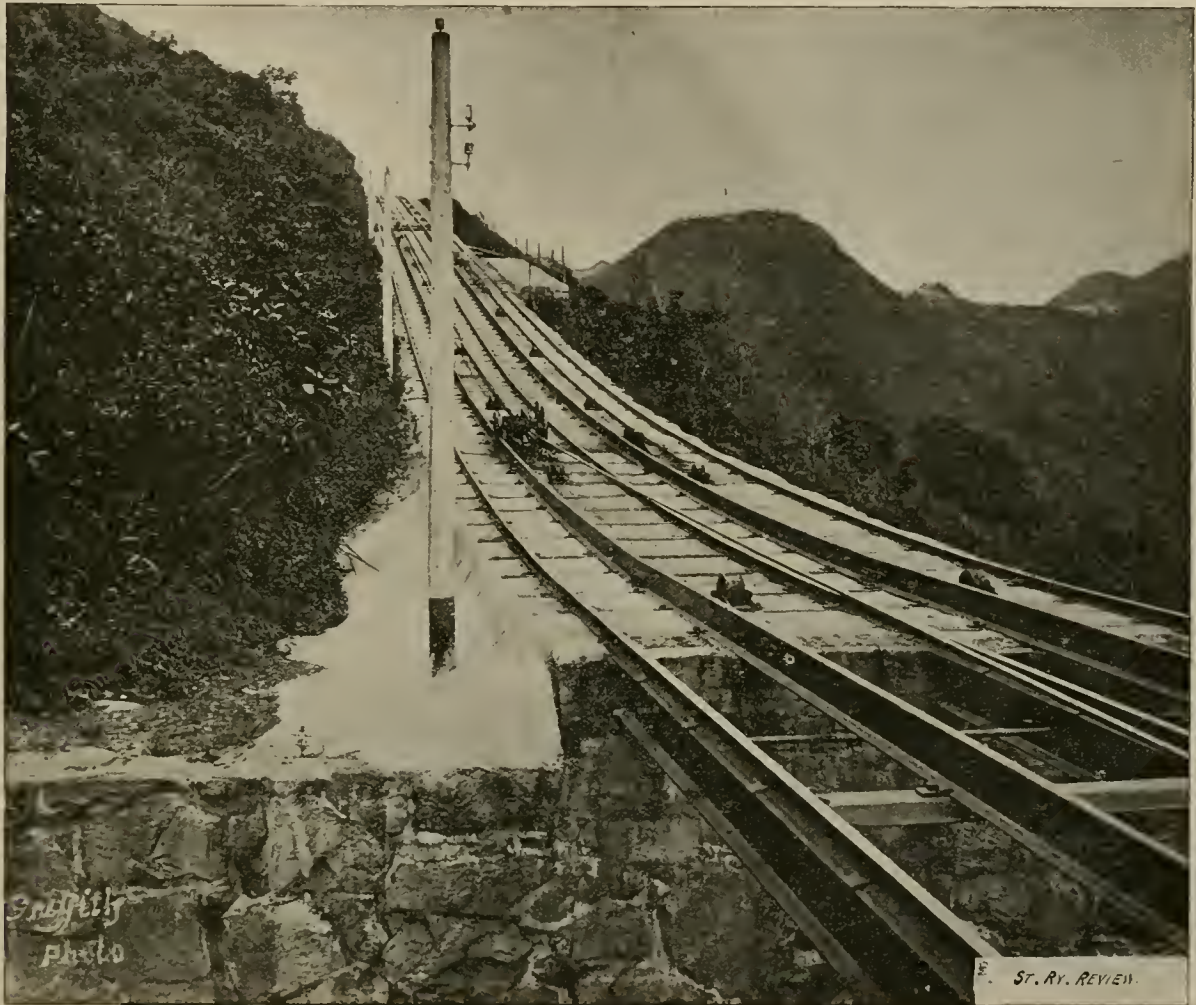
HONG KONG CABLE RAILWAY—SHOWING DEPRESSION PULLEY.
