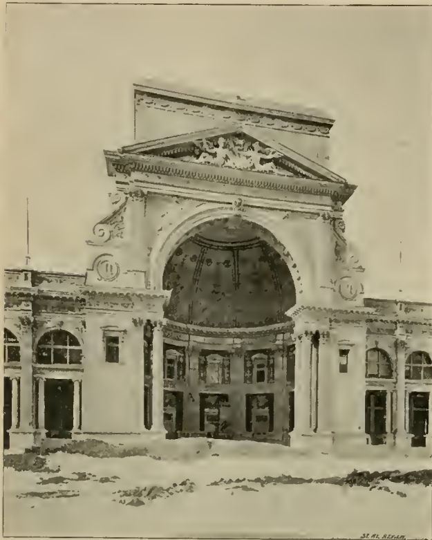
SOUTH ENTRANCE—ELECTRICAL BUILDING.
