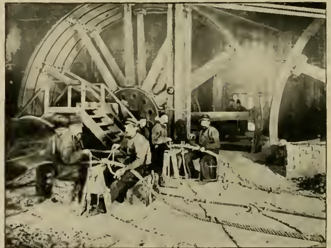
SPLICING THE TRANSMISSION ROPES.
