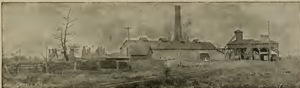
THE POWER STATION AT EDINBURG, ILL.
