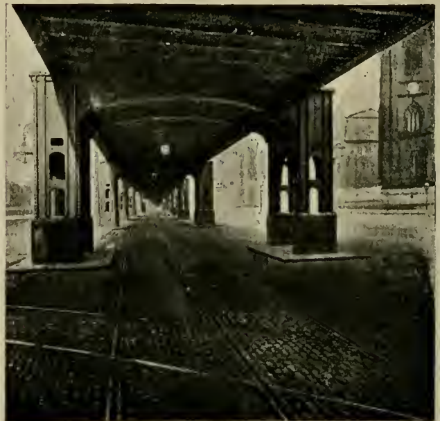
UNDER VIEW OF STRUCTURE.
