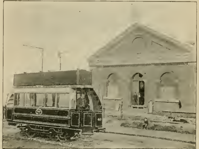
SOUTH STAFFORDSHIRE LINE.
