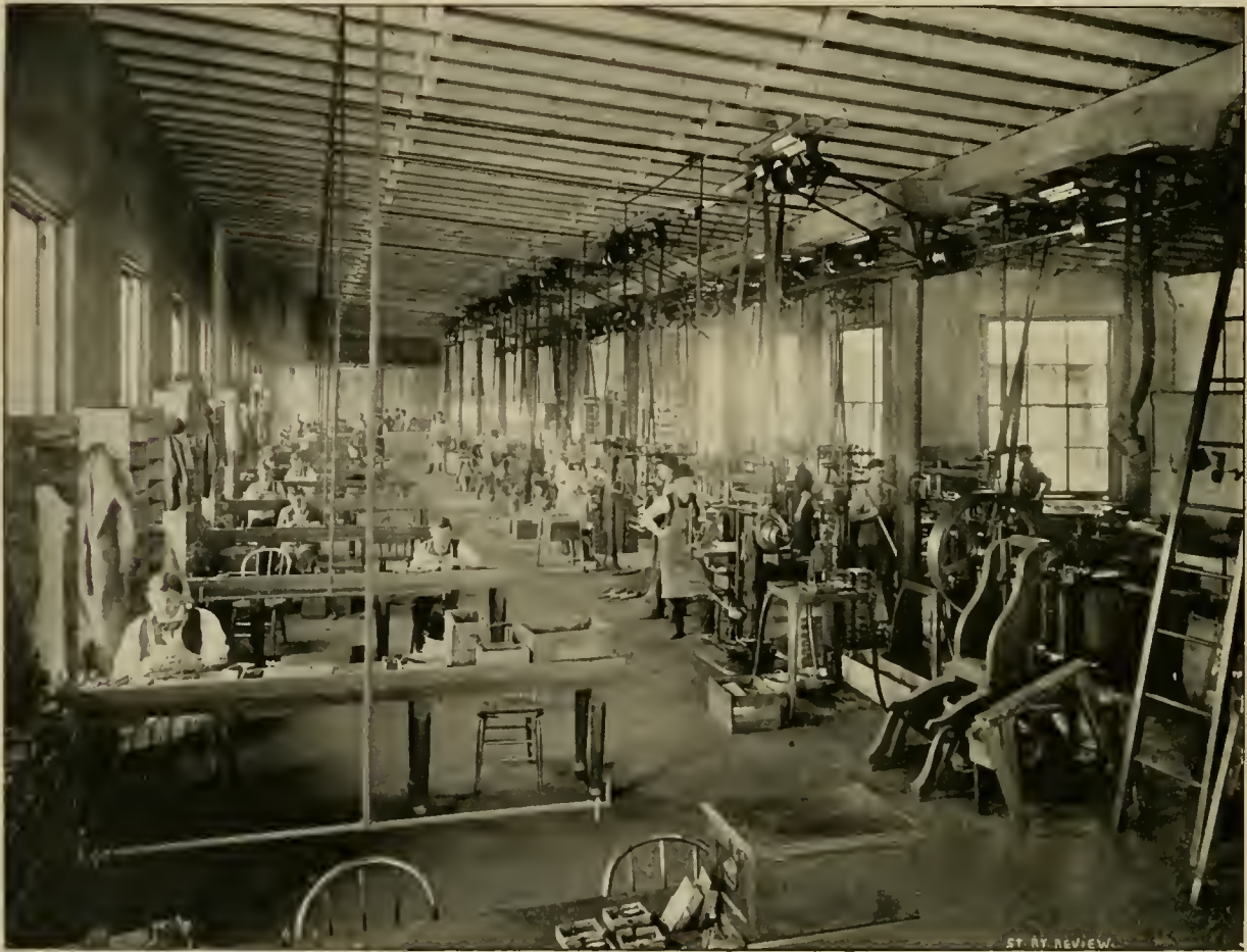
FACTORY SCENE IN THE WORKS OF THE MEAKER MANUFACTURING COMPANY, CHICAGO.
