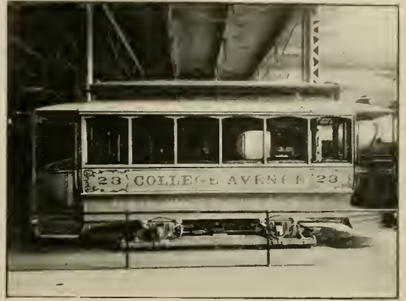
STEPHENSON ELECTRIC CAR.
