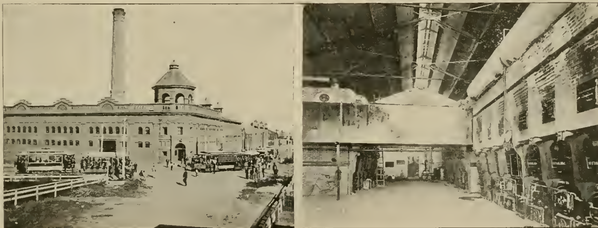
POWER HOUSE AND CAR BARN—BATTERY OF STIRLING BOILERS.
