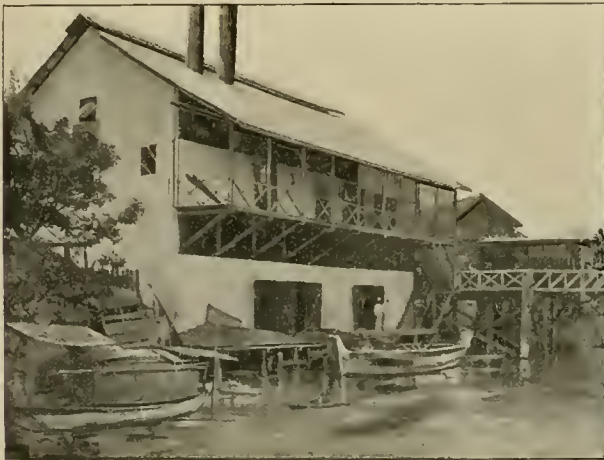
THE POWER HOUSE AT BANGKOK.
