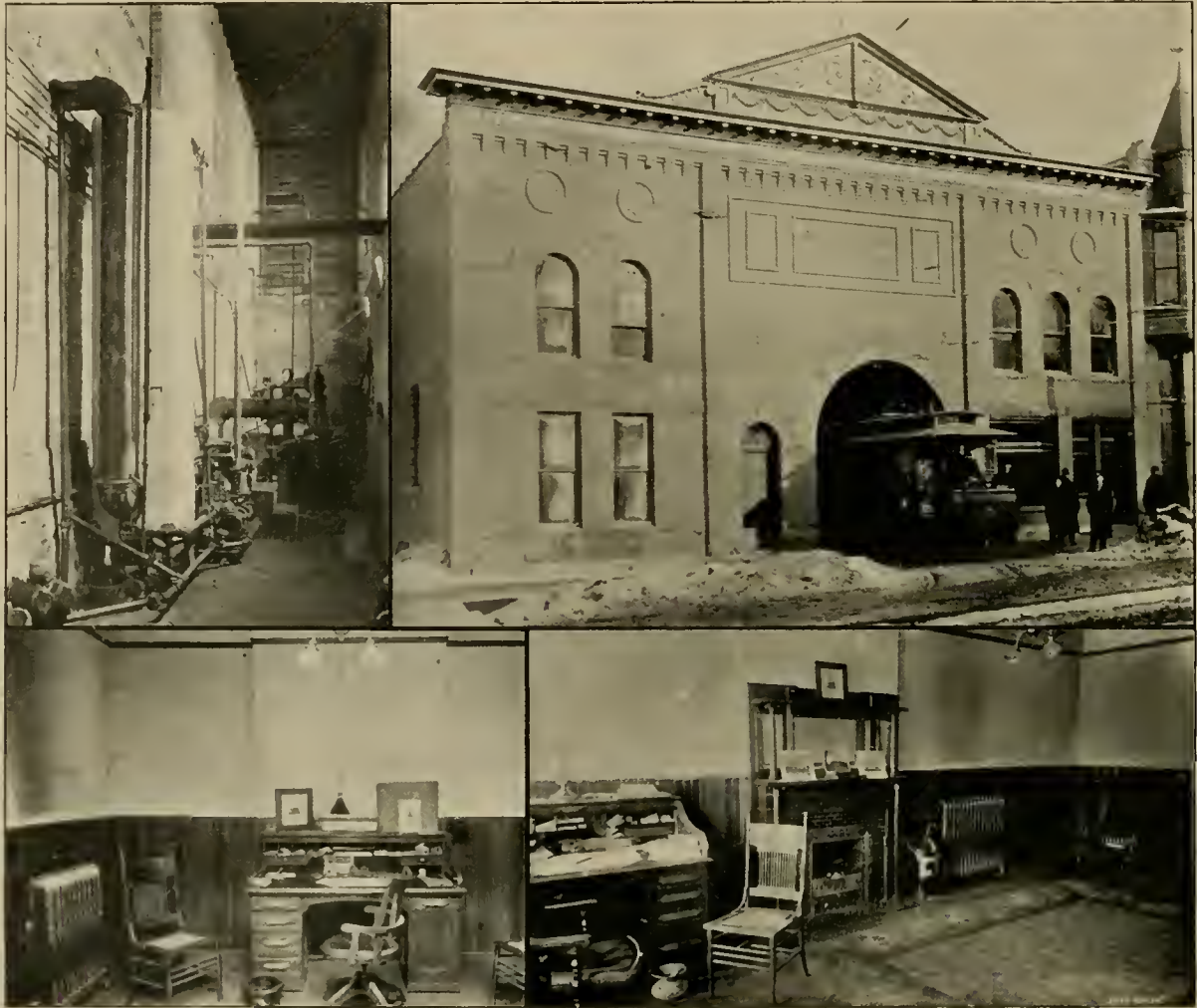
COLLES FEED WATER HEATER. ALLEN SHEWMAN'S OFFICE.
