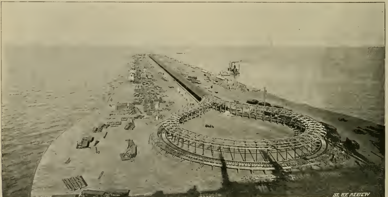
BIRD'S EYE VIEW OF PIER AND SIDEWALK FROM THE CASINO.
