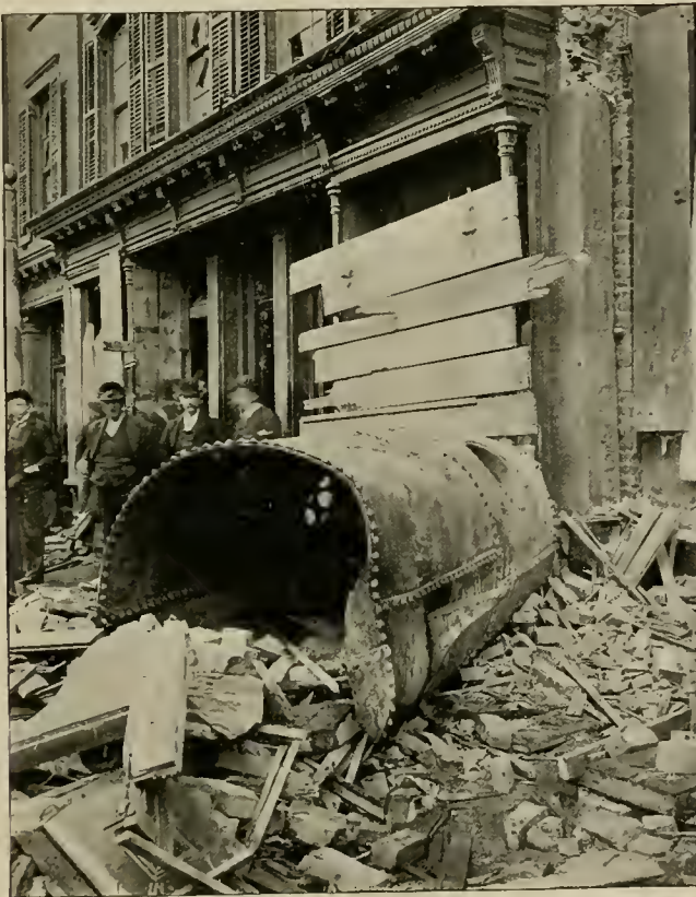
SOUTH END OF BOILER WHICH BLEW ACROSS THE STREET.
