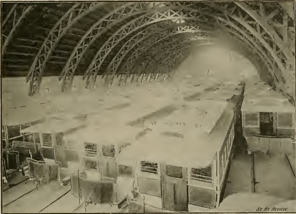
CAR HOUSE—MONTREAL STREET RAILWAY.
