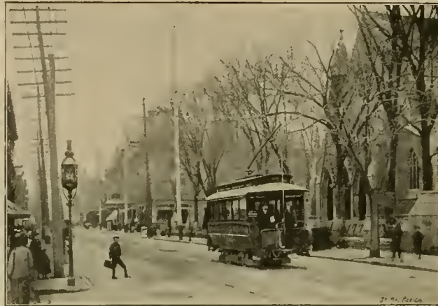
ST. CATHERINES STREET—LOOKING EAST.
