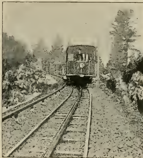
TRACK, COG AND CONDUCTOR RAILS.
