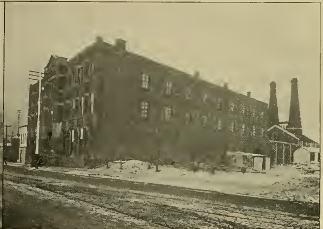
THE YOUNGSTOWN POWER STATION.
