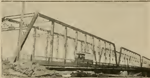
MAIN STREET BRIDGE.
