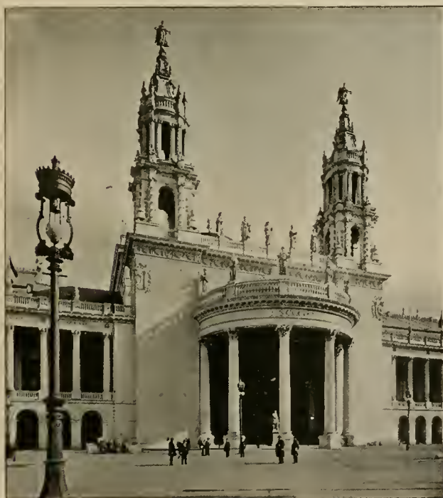
THE NORTH ENTRANCE TO MACHINERY HALL.
