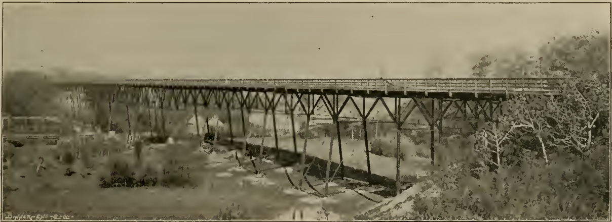
HIGH TRESTLE ON THE WAUWAUTOSA LINE.
