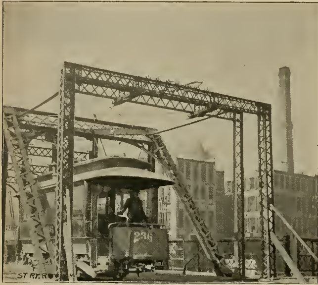
MICHIGAN STREET BRIDGE APPROACH.
