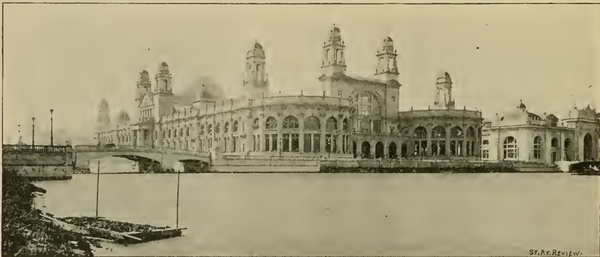
ELECTRICITY BUILDING. NORTH FRONT, VIEWED FROM THE NORTHWEST.
