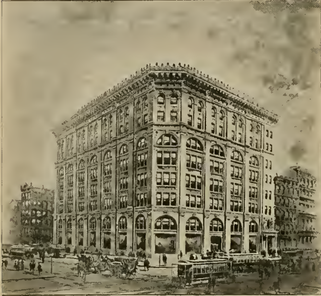
THE HOUSTON STREET POWER STATION.
