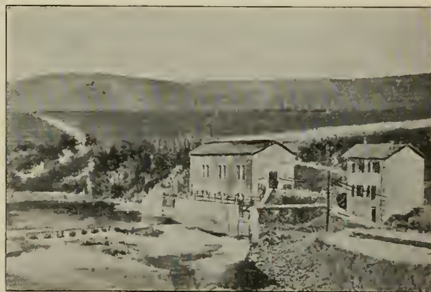
THE POWER STATION, SALEVE.
