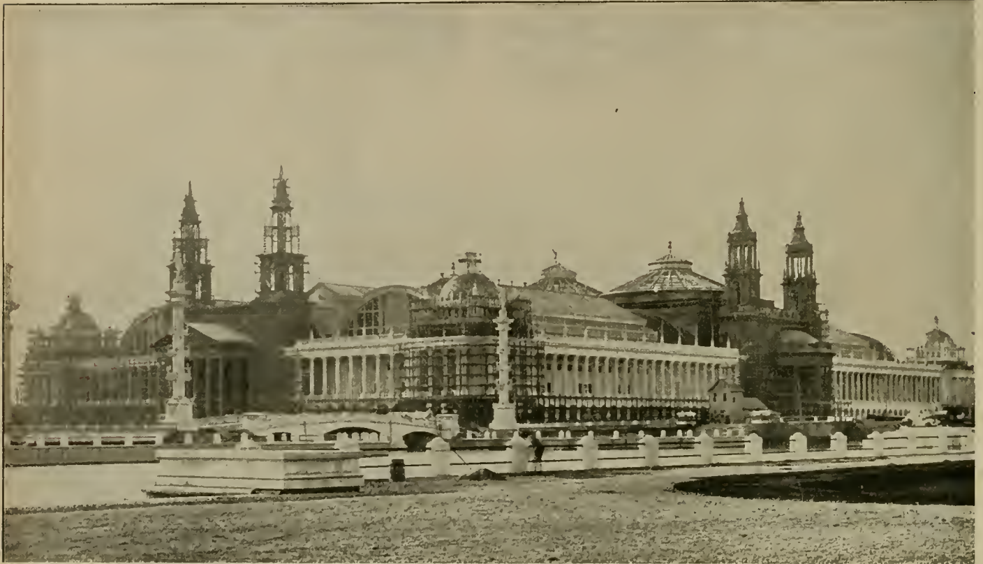
MACHINERY HALL — THE LAST IN EXTERIOR COMPLETION.
