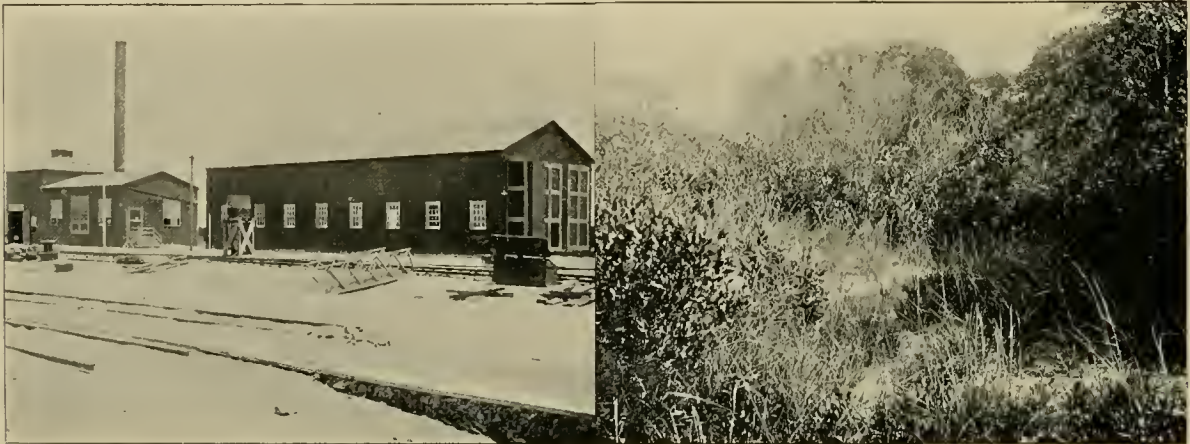
POWER HOUSE AND CAR BARN.
