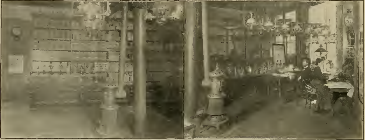
OFFICE AND GENERAL SALES ROOMS, SMITH FACTORY.
