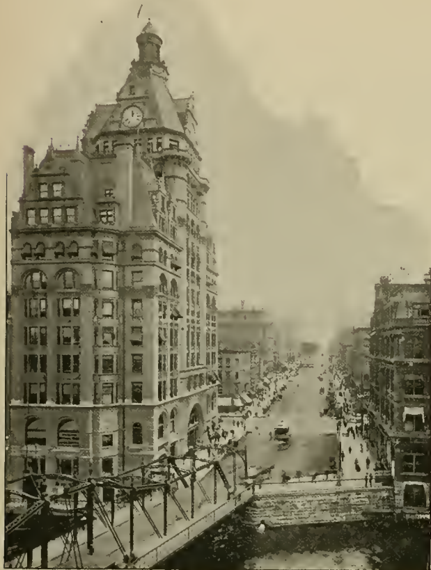
THE PABST BUILDING.
