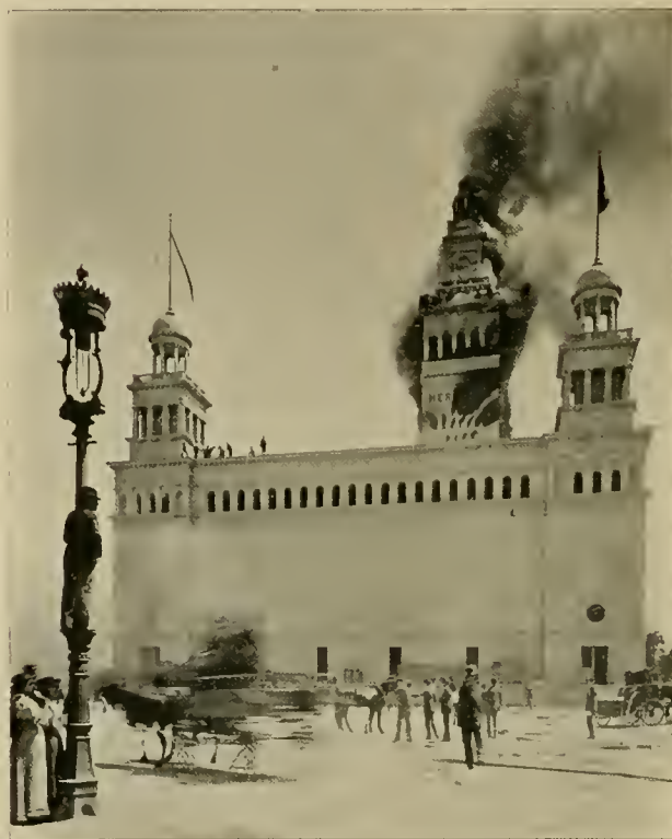
COLD STORAGE FIRE—INSTANTANEOUS PHOTOGRAPH AT MOMENT WHEN ESCAPE WAS DISCOVERED IMPOSSIBLE.
