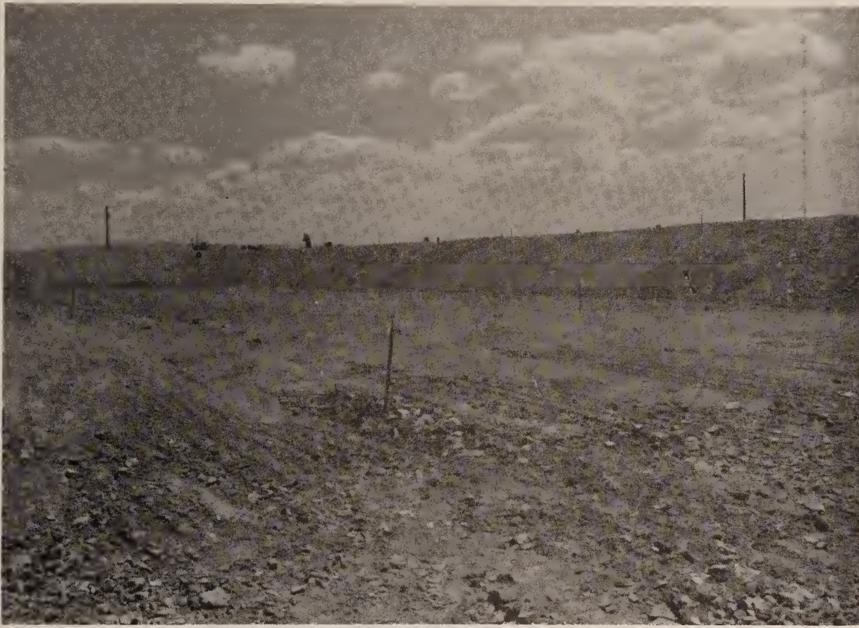
FIGURE 4-20a Pond C Construction Progress July 1979
