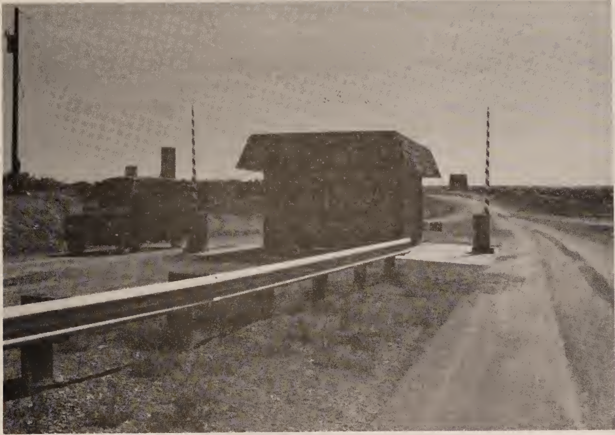
FIGURE 7-3 New Security Building on the Main Access Road - August 1979
