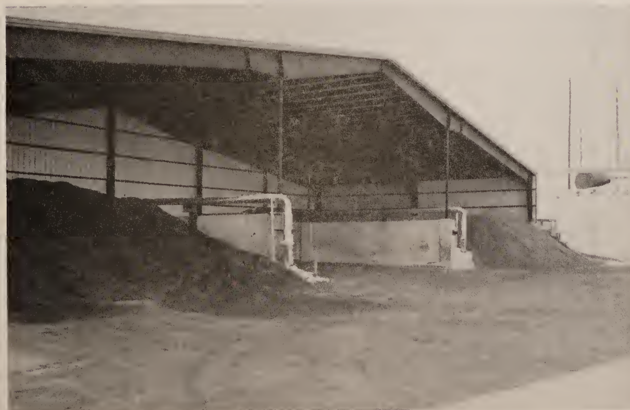
FIGURE 4-15 The Completed Aggregate Shelter - October 1979
