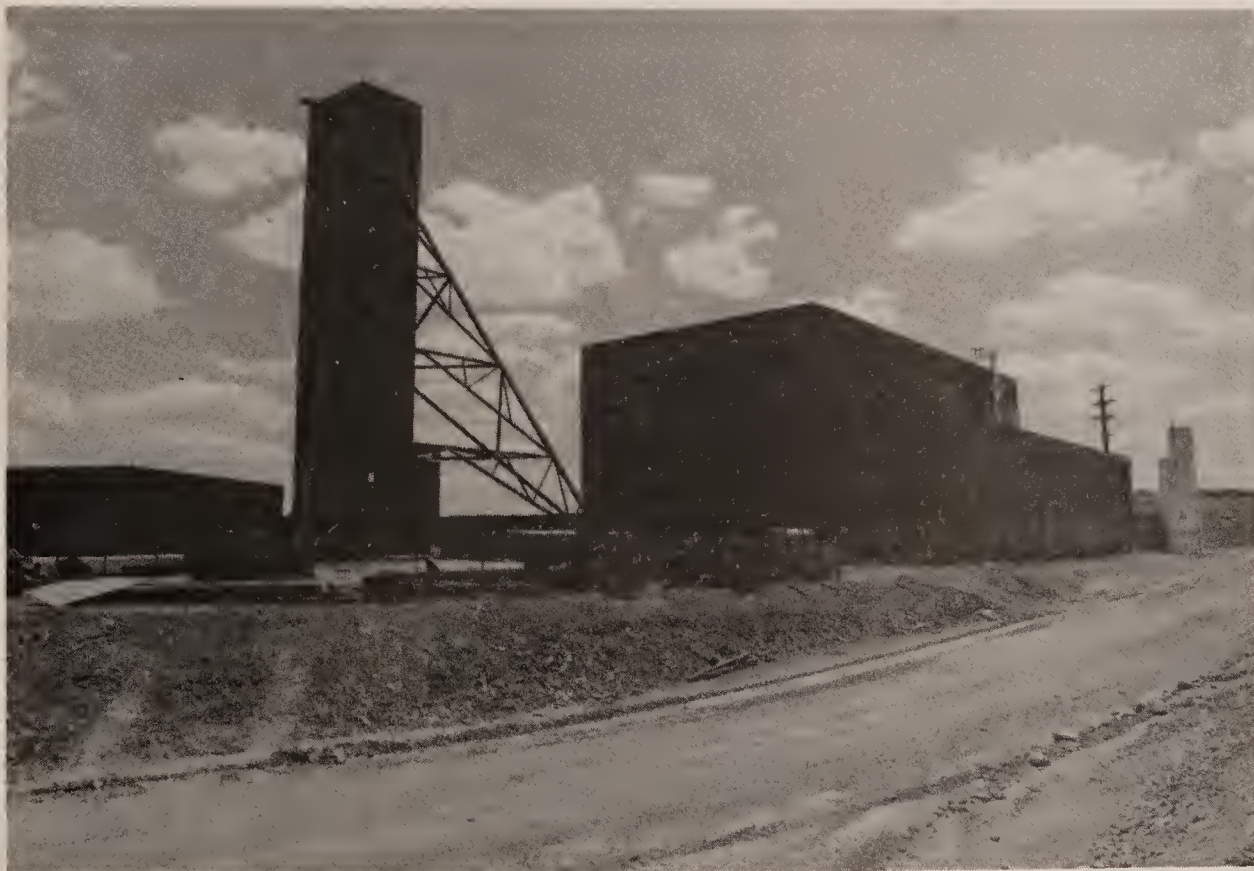
FIGURE 4-11 Exterior View of V/E Shaft and It's Hoist Houst - August 1979
