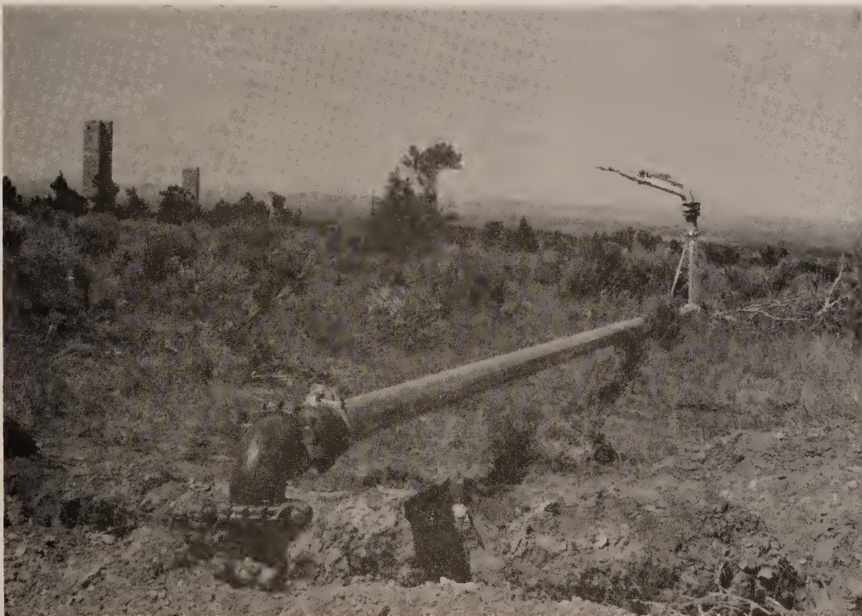
FIGURE 4-22b Sprinkler Irrigation System. Typical Sprinkler Head. August 1979
