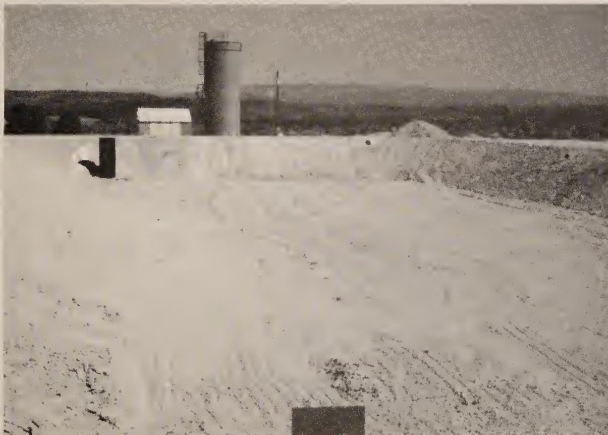
FIGURE 4-20b Pond C Progress - October 1979
