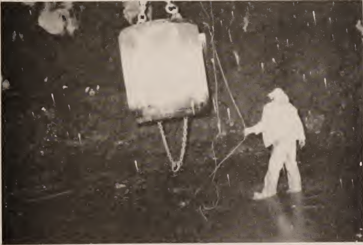
FIGURE 4-28 Production Shaft Bucket at Bottom of Shaft - November 1979
