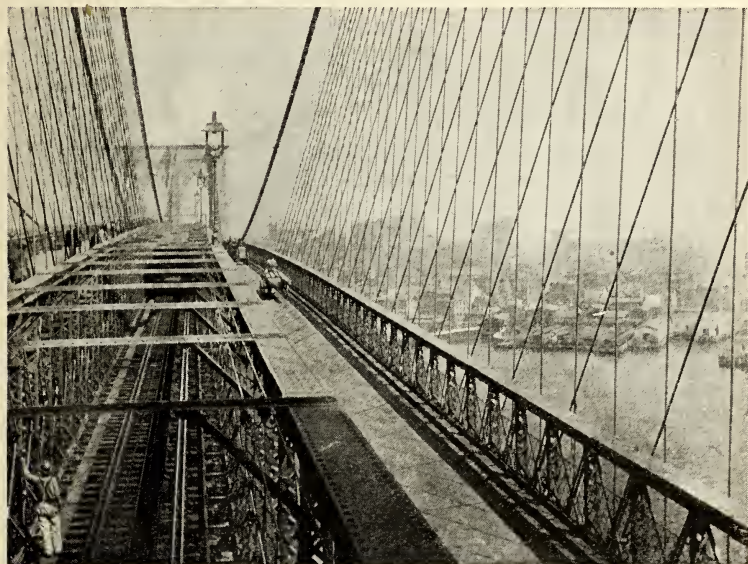
Railway and Driveway, South side.
