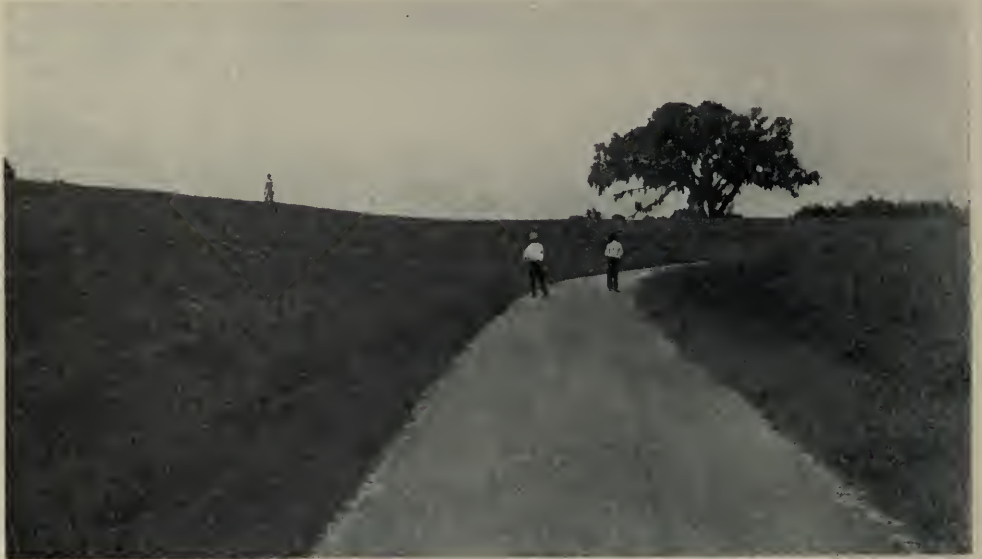
Adequate Levees Insure Protection from Future Floods
