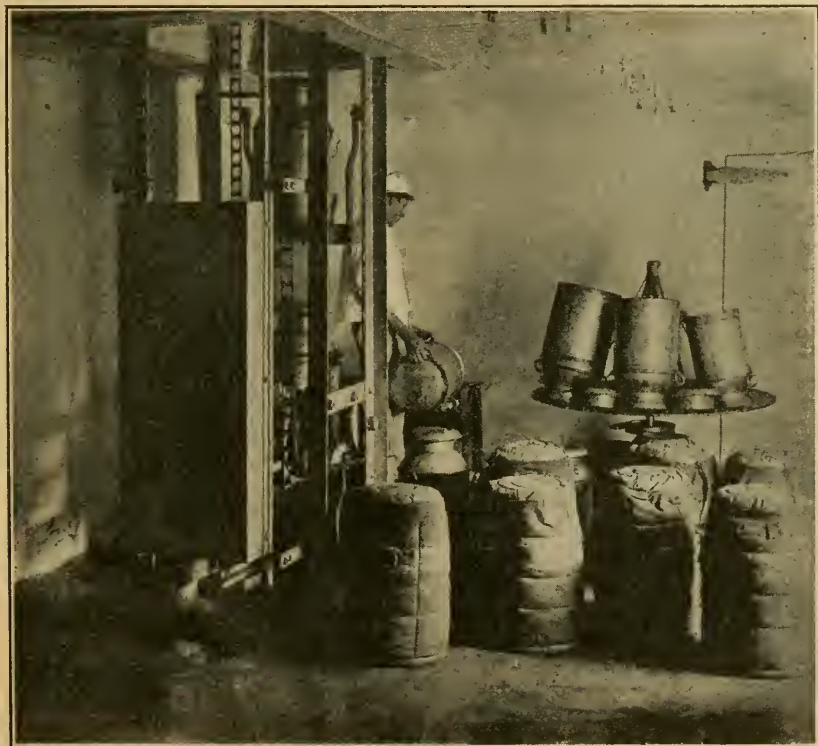
FIG. 2.—Method of draining cans to prevent waste. The illustration shows also jacketing of cans to keep milk cool.
