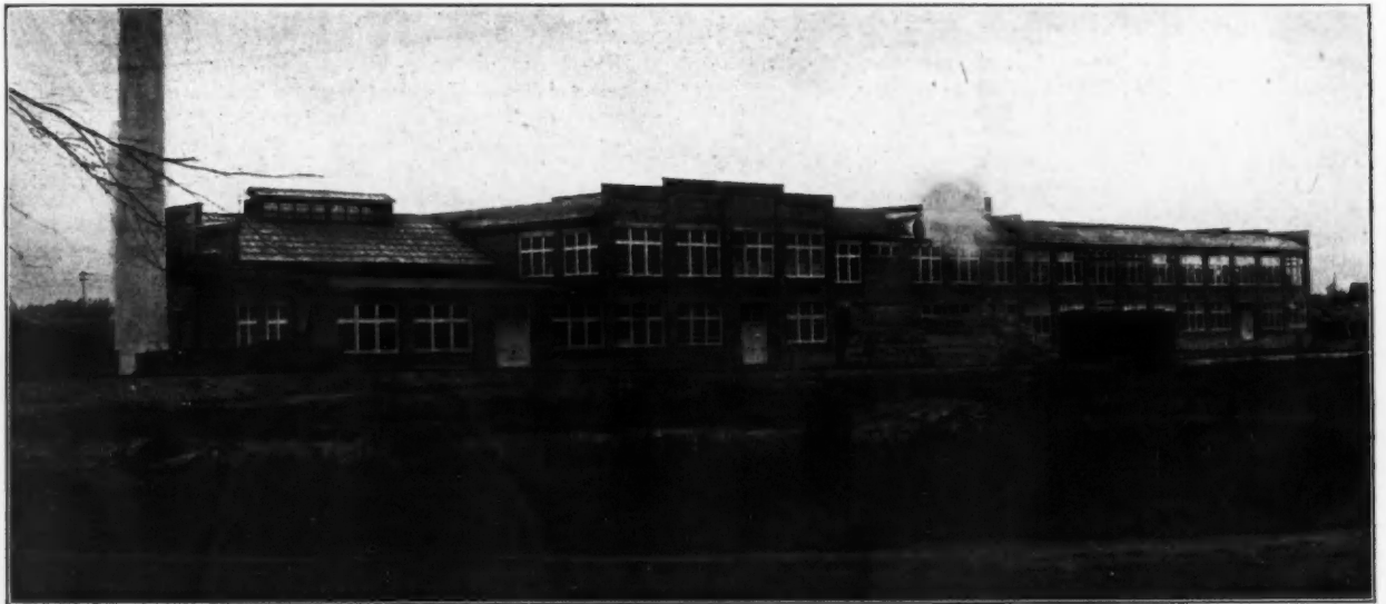
STEVENS POINT DIV. CONSOLIDATED WATER POWER & PAPER CO., STEVENS POINT, WIS.
