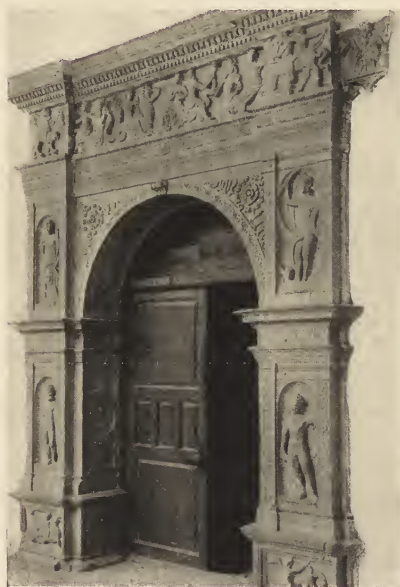
FIG. 103—Doorway in Upper Story of Patio, Castillo de Lacañahorra. By Michele Carlone of Genoa, 1508-12.
