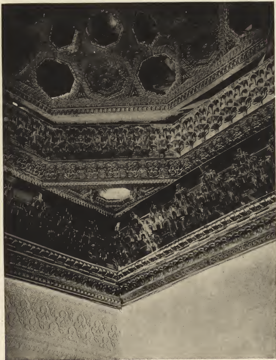
DILAPIDATED ARTESONADO IN A SMALL SALON OF THE PALACIO DE PEÑARANDA DE DUERO.
