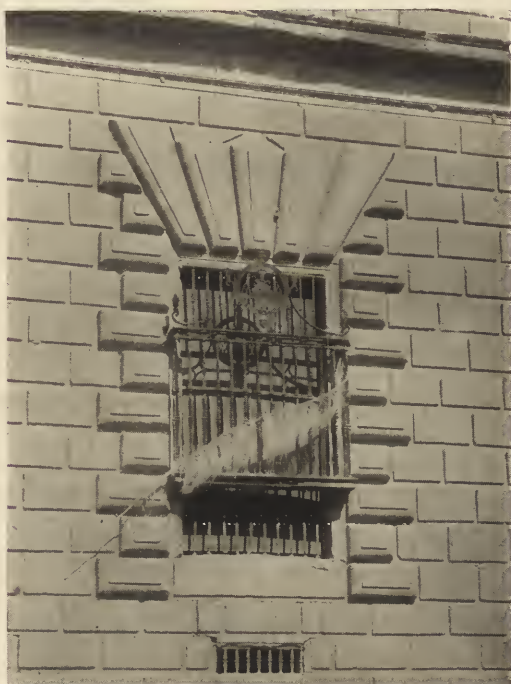
FIG. 130—Window in the Hospital de San Juan Bautista, Toledo.
