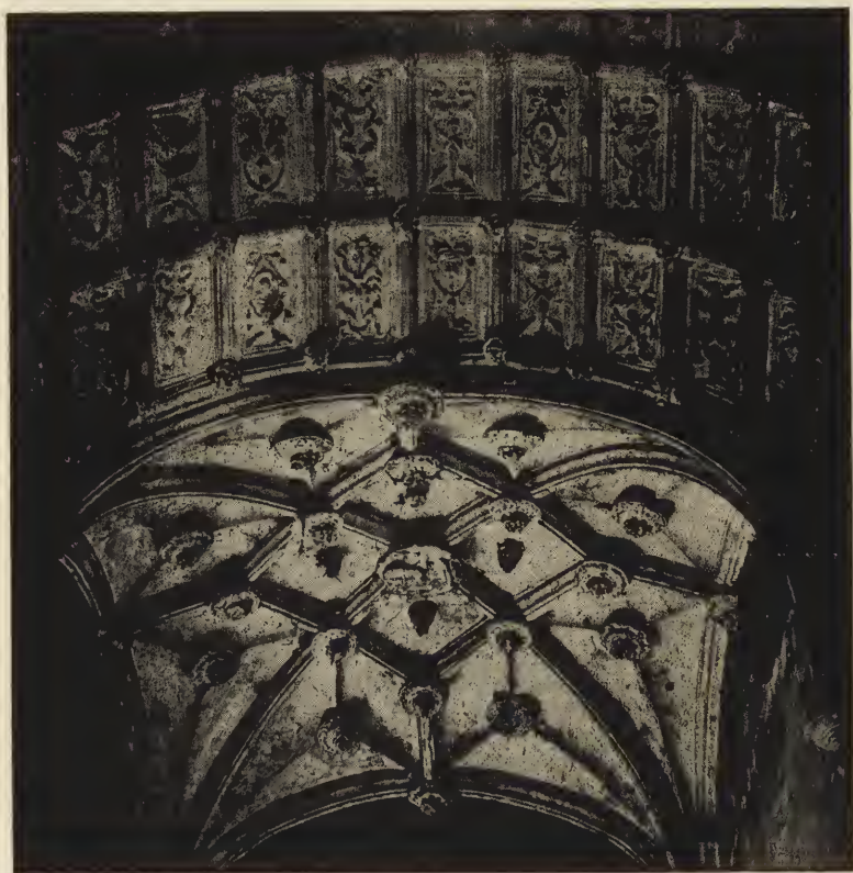
FIG. 31—Vaulting of Stairway in the Casa Miranda, Burgos. 1543.
