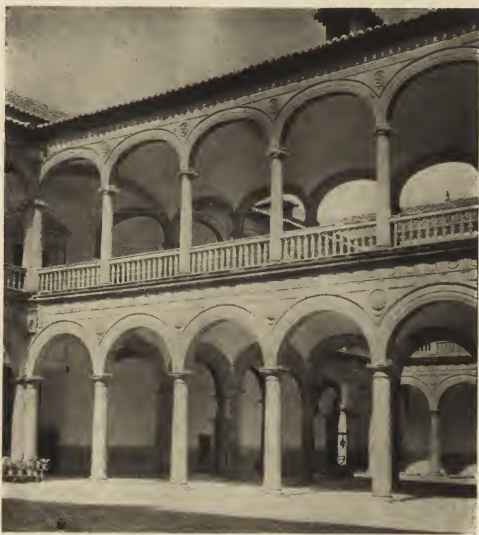
FIG. 129—Arcade Between Two Patios of the Hospital de San Juan Bautista (Afuera), Toledo.
