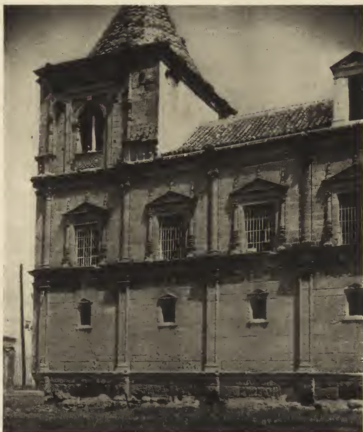
FIG. 134—Hospital Provincial (de la Sangre), Seville. Martin Gainza and Hernán Ruiz, Architects, 1559 et seq.
