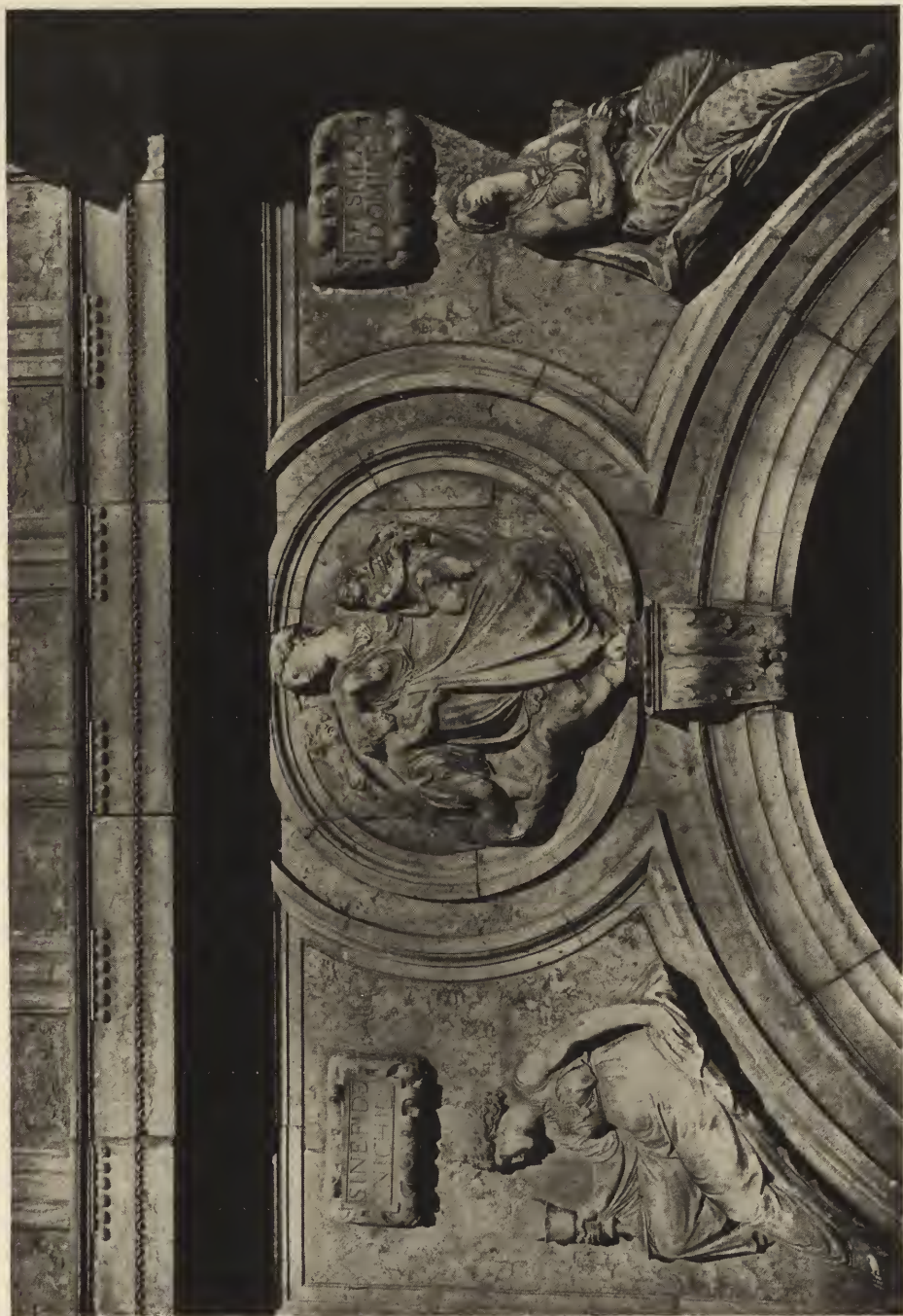
SPANDREL OVER MAIN PORTAL OF THE HOSPITAL PROVINCIAL, SEVILLE. Ascribed to Pietro Torrigiani.
