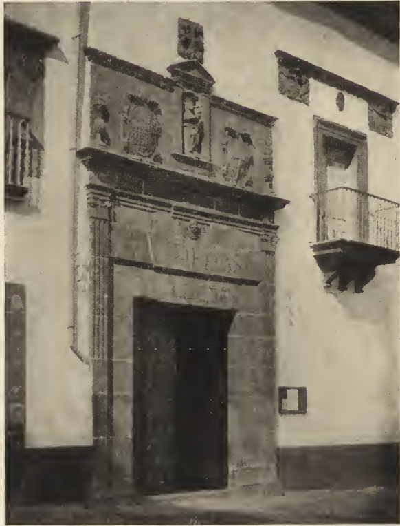
FIG. 60—Portal Adjoining the Bishop's Palace, Plasencia.
