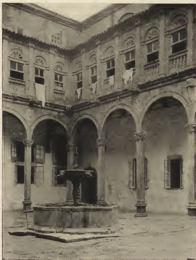
FIG. 8—Patio of the Hospital Real, Santiago de Compostela. Enrique de Egas, Architect, 1501-11.
