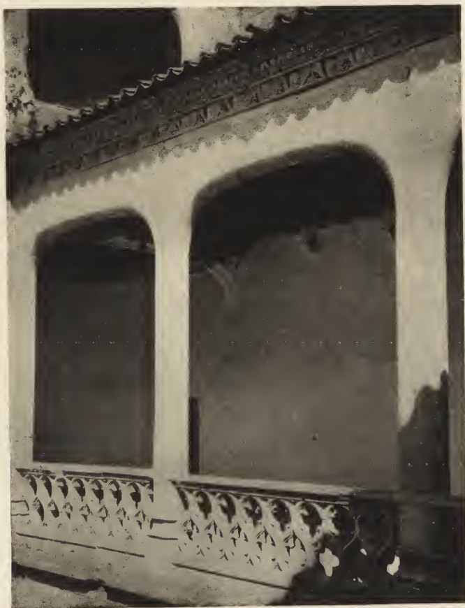
FIG. 52—Patio of the Castillo de Villanueva de Cañeda near Salamanca.
