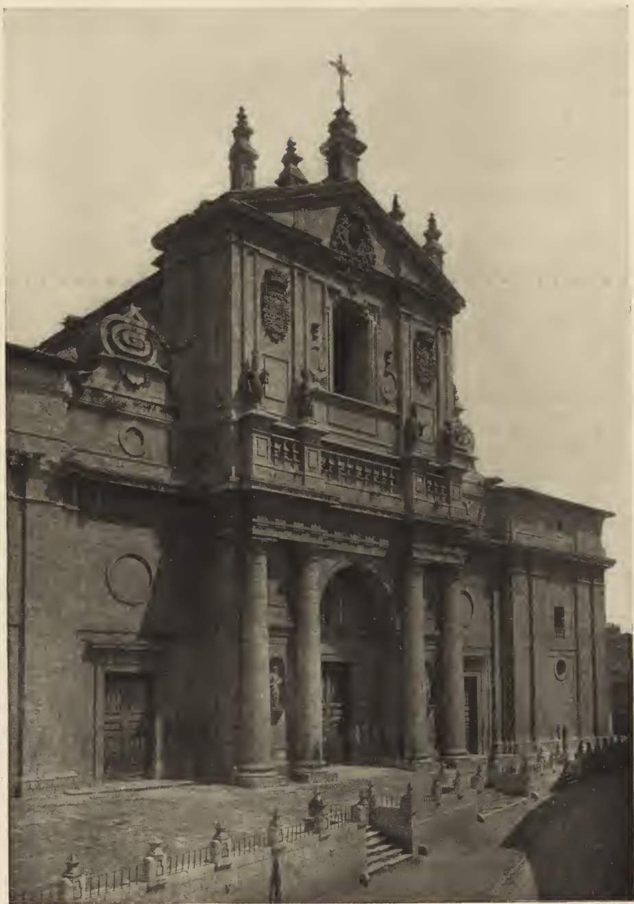
WEST FRONT OF THE CATHEDRAL OF VALLADOLID.
