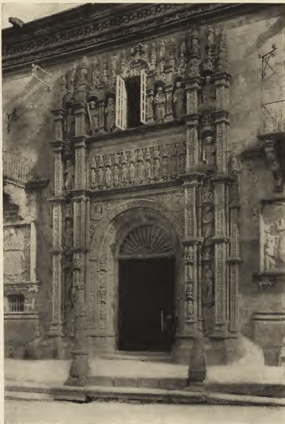
PORTAL OF THE HOSPITAL REAL, SANTIAGO DE COMPOSTELA. Enrique de Egas, Architect, 1501-11.
