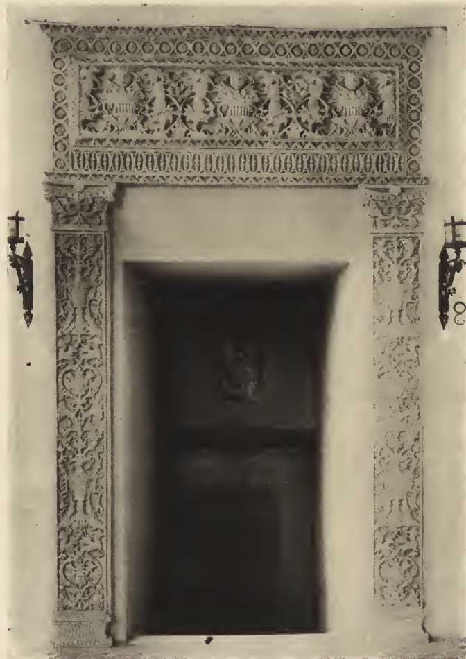
FIG. 82—Doorway in Upper Cloister of the Casa del Duque de Alba, Seville.
