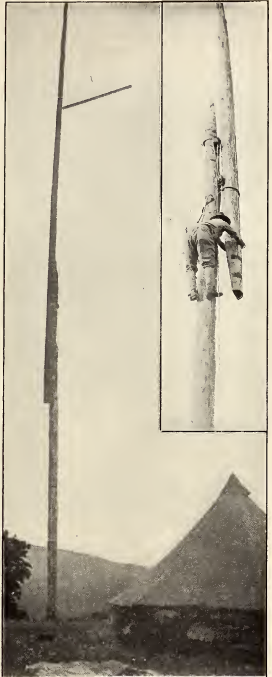
LOWER CUT: THE POLE AT WIRELESS STATION HEAD-QUARTERS. THE INSERTED CUT: MAKING THE JOINTS IN THE HEADQUARTERS WIRELESS MAST.
