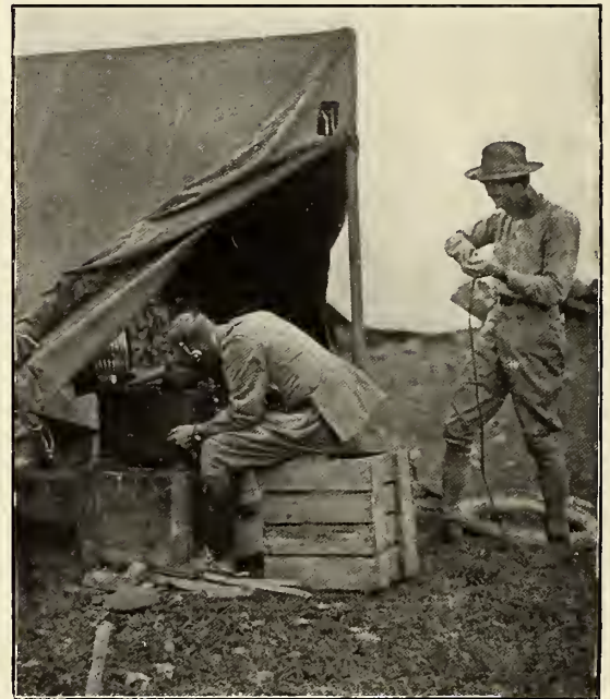
ERECTING A SEMI-PERMANENT WIRELESS SET.
