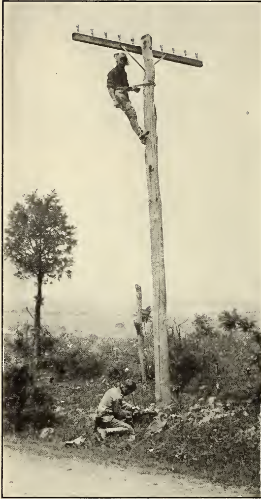
SENDING A MESSAGE ON A "STOLEN" WIRE. THE MAN AT THE TOP OF THE POLE IS WAITING TO DISCONNECT THE WIRE.
