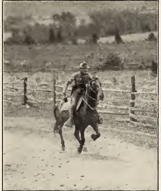
LAYING A BUZZER WIRE FROM A HAND-REEL, AT A GALLOP.
