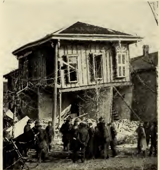
THE HOUSE THAT WAS CURIOUSLY WRECKED BY A GAS EXPLOSION.
