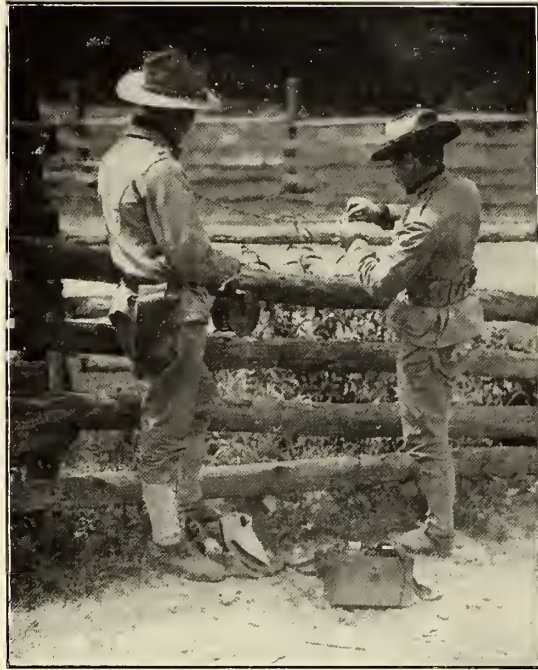
ATTACHING A BUZZER WIRE TO THE BARBED WIRE OF A FENCE. THE BUZZER KIT IS ON THE GROUND AND THE REEL OF WIRE IN THE HAND OF THE SOLDIER AT THE LEFT.
