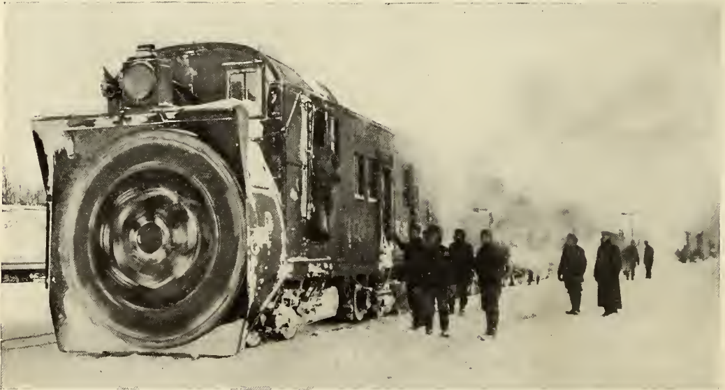
READY TO "BUCK" A DRIFT. NOTICE THE WHIRLING BLADES.
