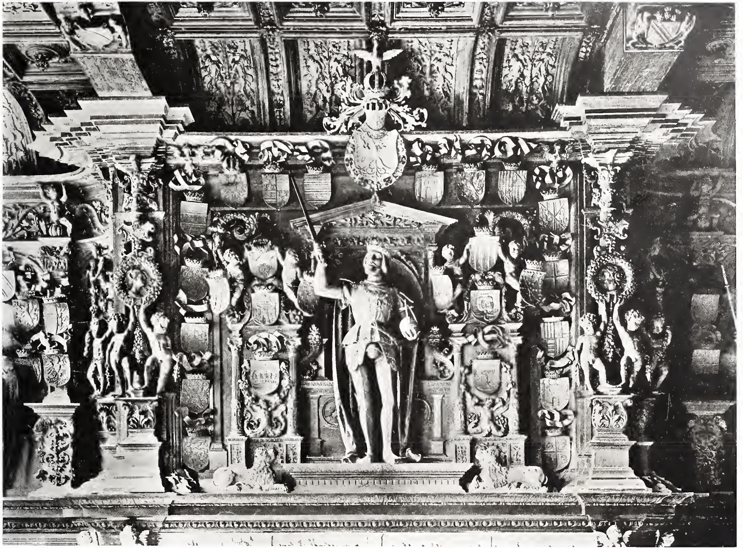
CHIMNEY-PIECE IN THE COUNCIL CHAMBER OF THE HOTEL OF THE LIBERTY OF BRUGES. DESIGNED BY LANCELOT BLONDEEL
