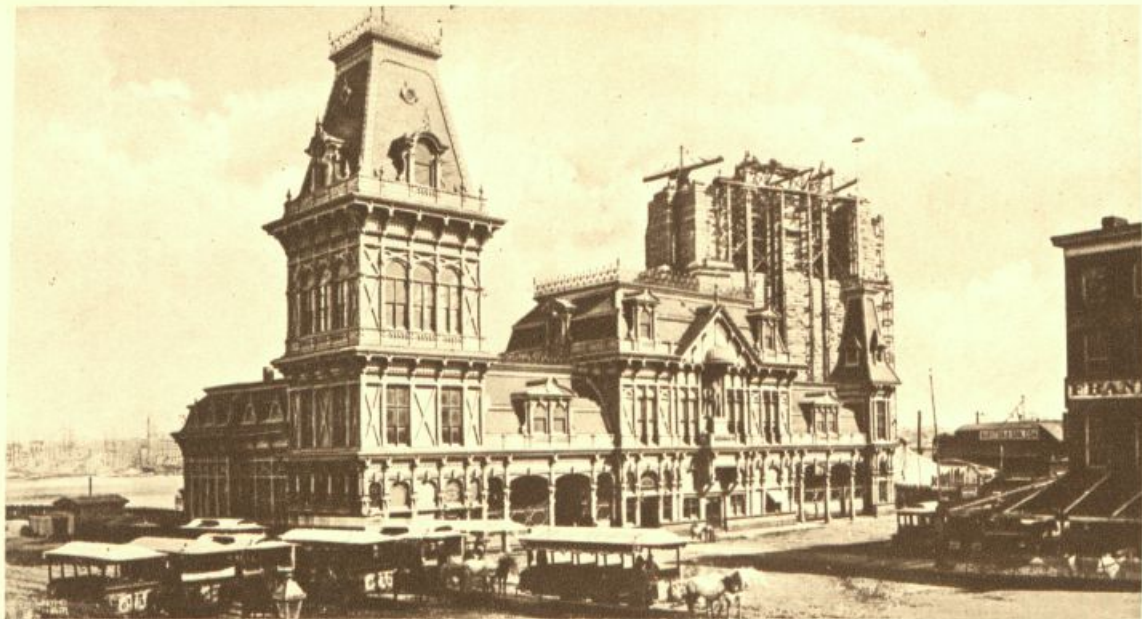
Fulton Ferry House, Brooklyn, 1874. At this time, the main artery of travel between New York and Brooklyn. Tower of the Brooklyn Bridge at right, in course of construction.
