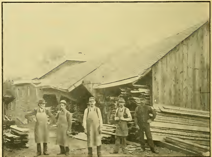
Borrowed Photo. JACOB RUSH'S SASH AND BLIND FACTORY AND PLANING MILL.
