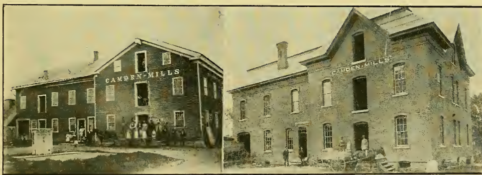
PENFIELD & STONE'S FLOUR AND FEED MILL.
