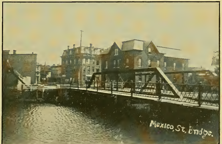
MEXICO STREET BRIDGE.
