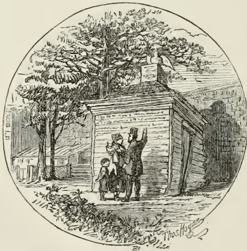
THE PRESENT CONDITION OF THE ‘MARTYRS’ MONUMENT.’”
