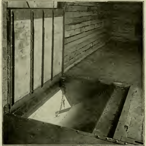
Interior of Canadian Pacific Box Car Showing Grain Door and One Open Hopper.
