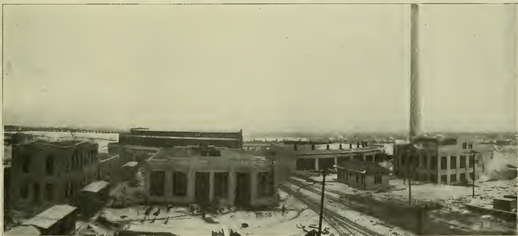
General View of Locomotive Group.
