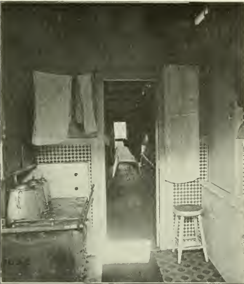
Kitchen and Dining Car Used in Wrecking Trains on the Erie.
