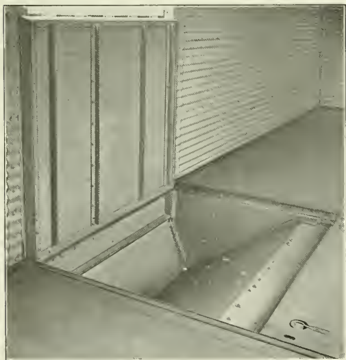
Hopper Bottom in Connection with Metal Sheathing.
