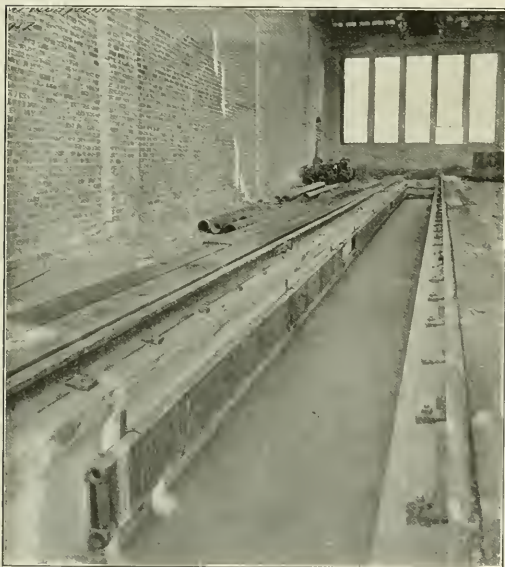
Typical Engine Pit.
