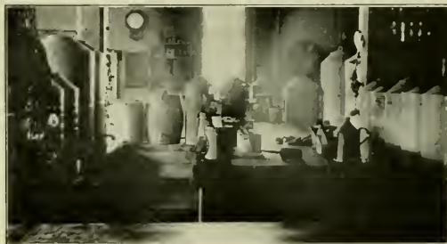
Store Room in the Paint Shop.
