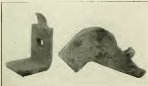
Two Parts of a Coach Truck Transom After Being Formed with Dies Under a Steam Hammer.
