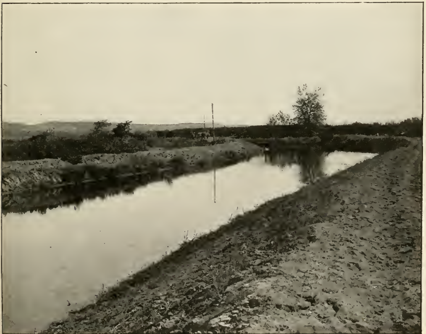
b. Along the line of Sunnyside Canal, Washington.
