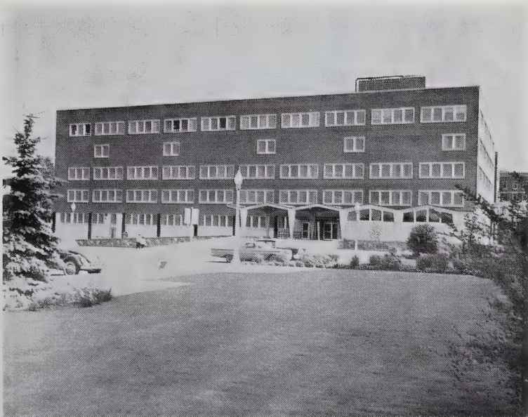
Clinical Services Building at the University of Alberta Hospital in Edmonton showing the emergency entrance.
