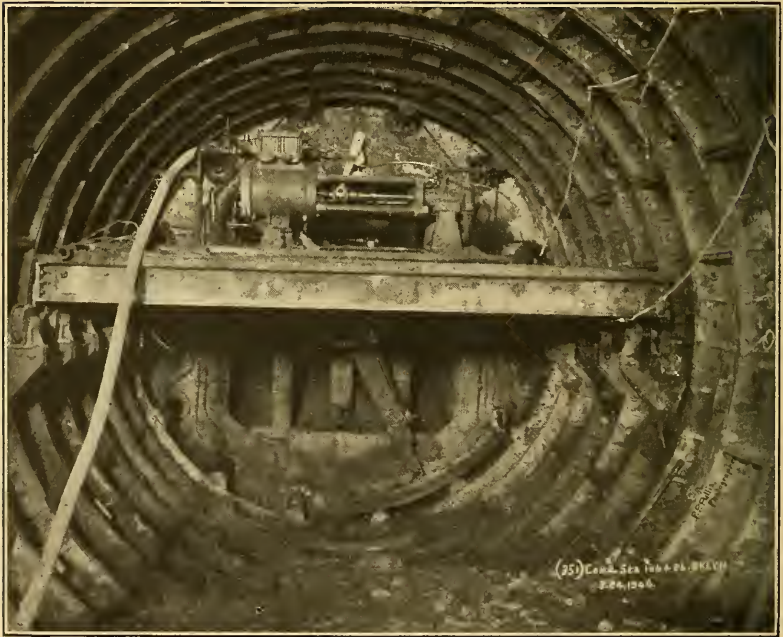
SUBWAY: SHIELD IN EAST RIVER TUNNEL.
