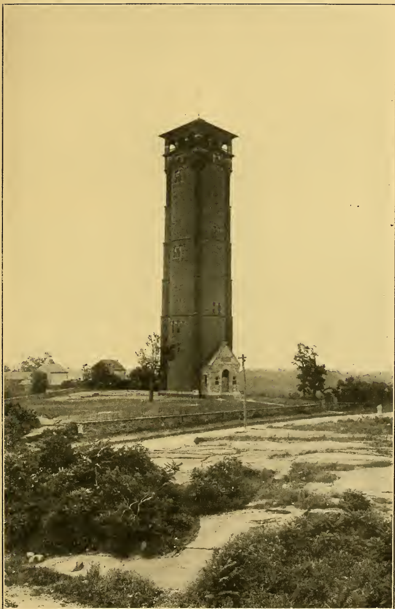
ELM STREET WATER TOWER, YONKERS.
