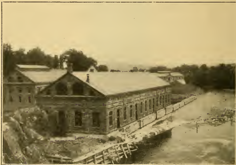
LITTLE FALLS PUMPING STATION.
