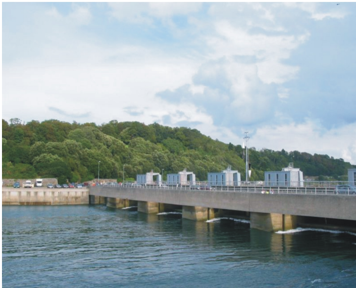
Figure 7: Dam of the tidal power plant on the estuary of the Rance River, Bretagne, France
