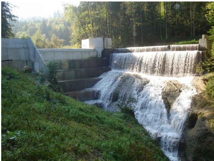
Figure 6: Small hydropower plant, Buchholz, Switzerland.
