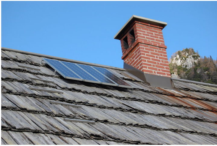
Figure 5: An example of solar power, using solar cells to convert sunlight into electricity.
