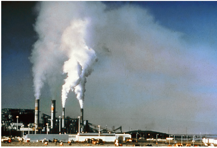
Figure 3: A major source of air pollution is the burning of fossil fuels from factories, power plants, and motor vehicles. Photo was taken prior to installation of emission controls equipment for removal of sulfur dioxide and particulate matter.
