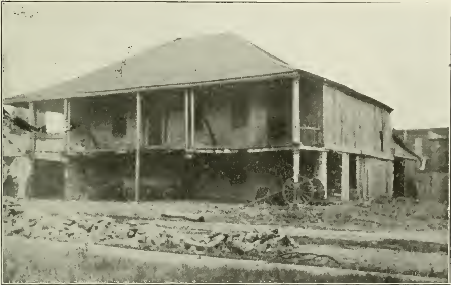
OLD GOVERNMENT BUILDING, FORT SCOTT
