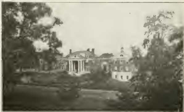
UNIVERSITY HOSPITAL BUILDINGS.
