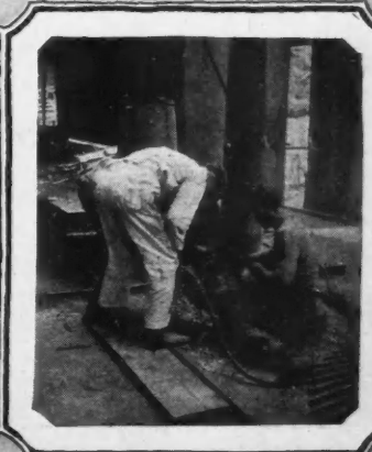
Repairing a Gyratory Crusher
