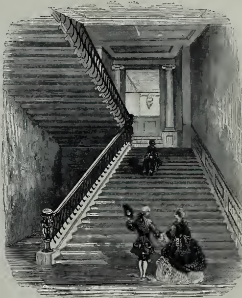
STAIRCASE IN SIR JOSHUA REYNOLDS'S HOUSE, LEICESTER-SQUARE.
