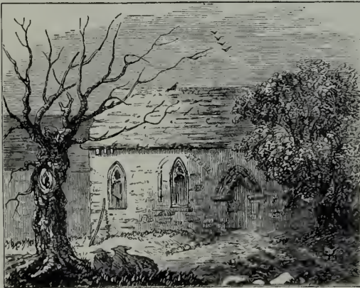
CRESLOW CHURCH, NORTH SIDE.
