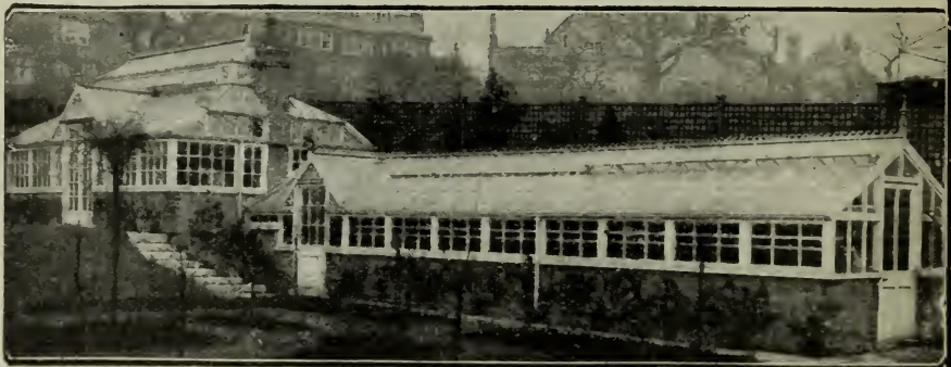
ERECTED AT HAMPSTEAD.
