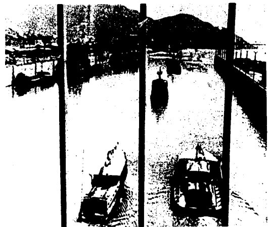
FIGURE 18. Iron Gate project. Near site of recently opened lock on Romanian shore of Danube. (U/OU)
