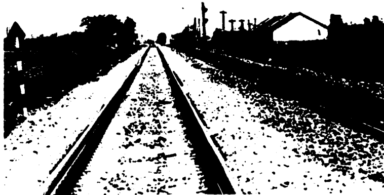
FIGURE 15. Double-track railroad section between Ploiești and Buzău. Newly renovated track with welded rail, prestressed reinforced-concrete ties, and crushed rock ballast alongside older track (right) with wooden ties. (C)
