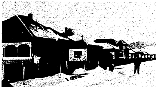
FIGURE 35. Newly constructed village housing in Otlenia, southwestern Romania (U/OU)
