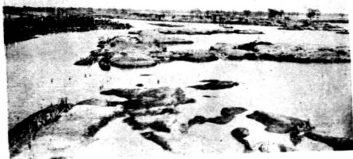
擋廟西堤全部堵合後之鳥瞰 ★
