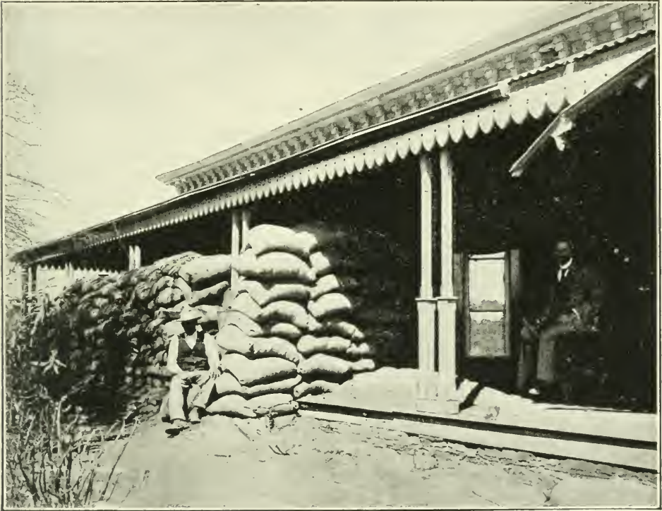
THE SIEGE OF KIMBERLEY: TYPICAL SPLINTER-PROOF SHELTER OF SAND-BAGS AND IRON PLATES
