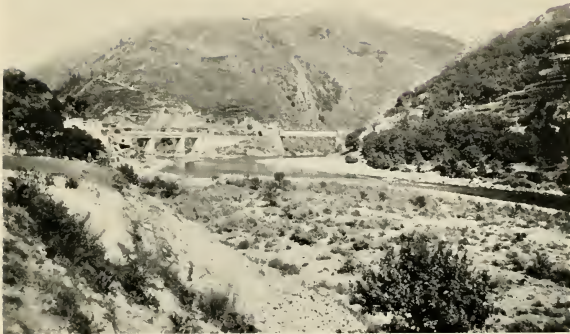
LOS PEARES, SHOWING THE RAILWAY BRIDGE ACROSS THE MIÑO.
