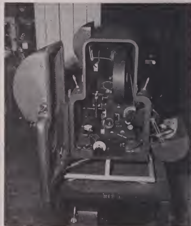
END VIEW of the Natural Vision 3-D motion picture camera in blimp. Unit consists of two Standard Mitchell 35mm NC cameras mounted opposed, with lenses picking up image from angular mirrors.
