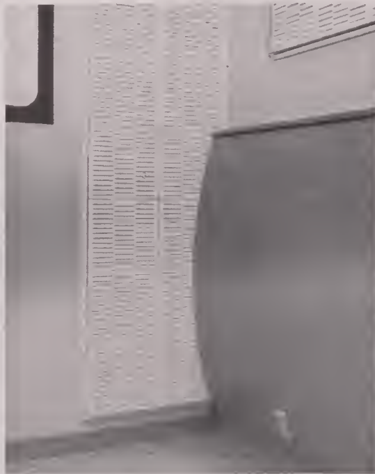
POLYCYLINDRICAL diffuser panels up front fill dual role of absorbing low-frequency energy and diffusing reflected sound.
