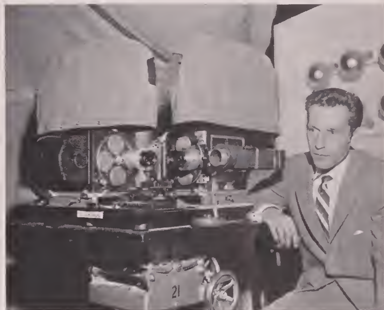
MGM's 3-D camera design follows radical departure in that two Mitchell 35's are mounted at right angles. Only one mirror is used. Because of several innovations, extreme closeups in perfect rendition are claimed for the camera, which is being inspected here by MGM executive, Arthur Loew, Jr.
