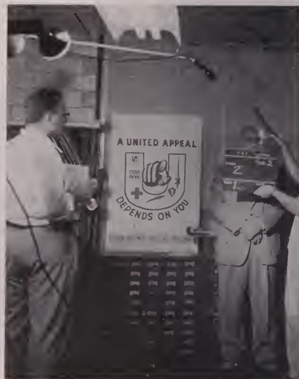
USE OF CLAPSTICK and slate makes it easy to put sync marks on both picture and sound films. These are matched up in editing to insure synchronization.
