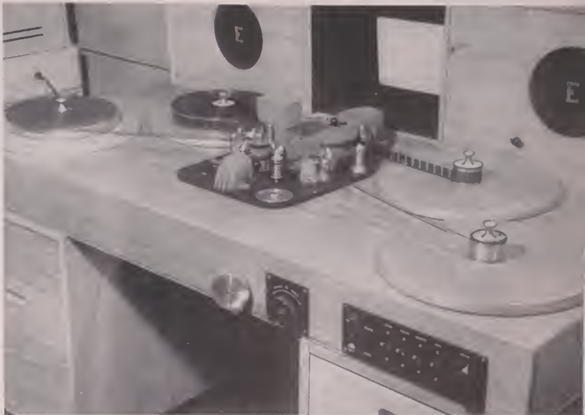
Fig. 1—The Precision Film Editor, with 7" x 9" viewing screen.
