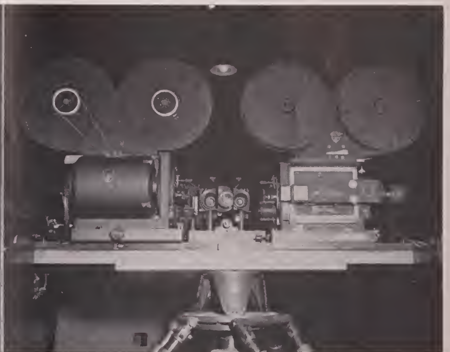
VIEW of Natural Vision 3-D camera with blimp removed. Here may be seen the two divergent mirrors in center and the front element of the central viewfinder set between them. Camera features a fixed interaxial and variable parallax control.
