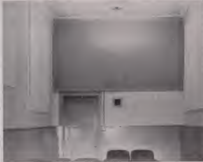
VIEW TOWARD rear of some room. Note that greater part of rear wall surface is covered with plywood diffusing elements that receive and properly treat sound energy.
