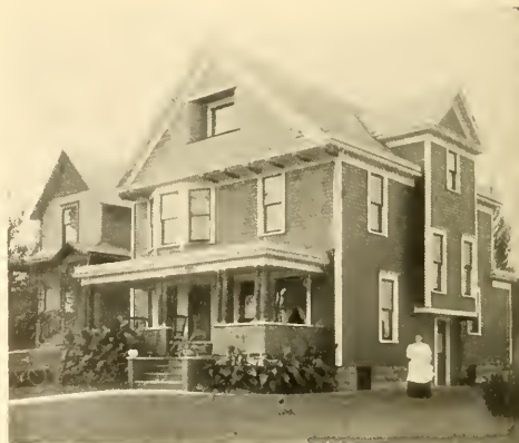
RESIDENCE OF ELMER A. GAULT, AKRON
