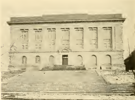
NEW COURT HOUSE, AKRON
