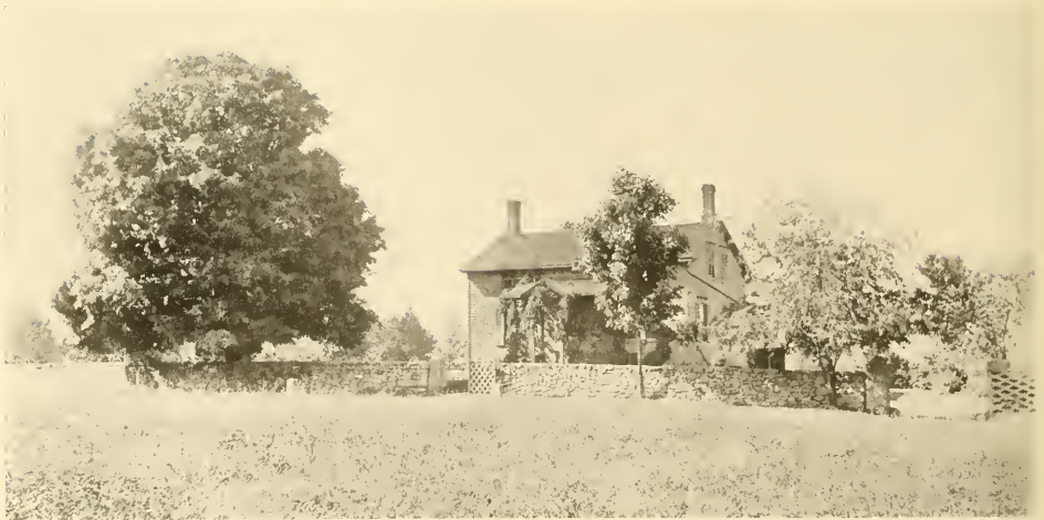
THE OLD JOHN BROWN HOME BEFORE BEING REMODELED
