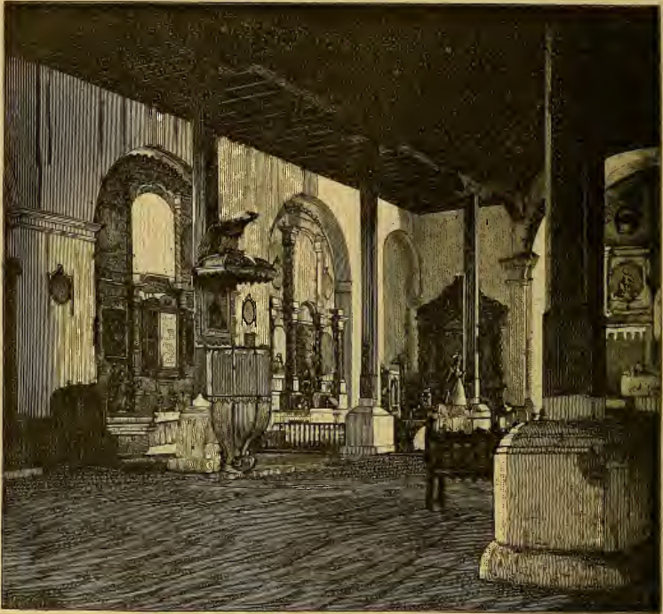
Interior of the Church at Coban.
