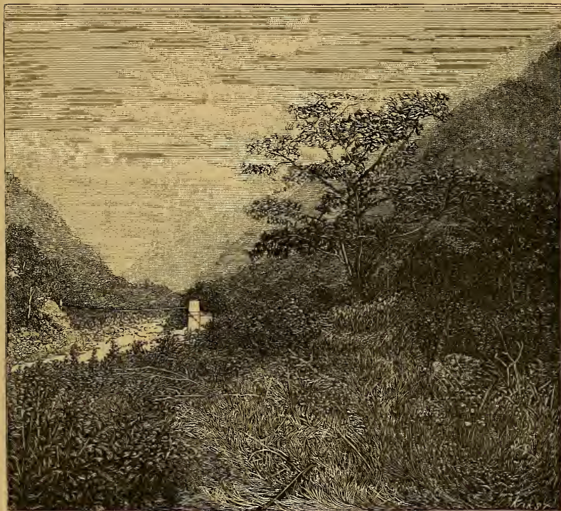
Rope Bridge over the Chixoy.
