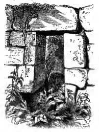
at top, where they are covered by a massive lintel, 3 feet 5 inches long, which spans the entire wall. The inner faces of the jamb stones are smooth, as at Killursa.
