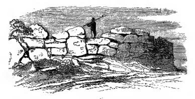
walls of unhewn stone, of a whitish hue, from the lichens covering them, are 9 feet 4 inches thick, and, although lowered in many places, still average 7 feet 7 inches high.
