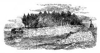
joined illustration, taken from the north-east. The wall of this fort, although not built of large stones, is 10 feet thick, and 6 feet high; its circumference is 393 feet. An outer
