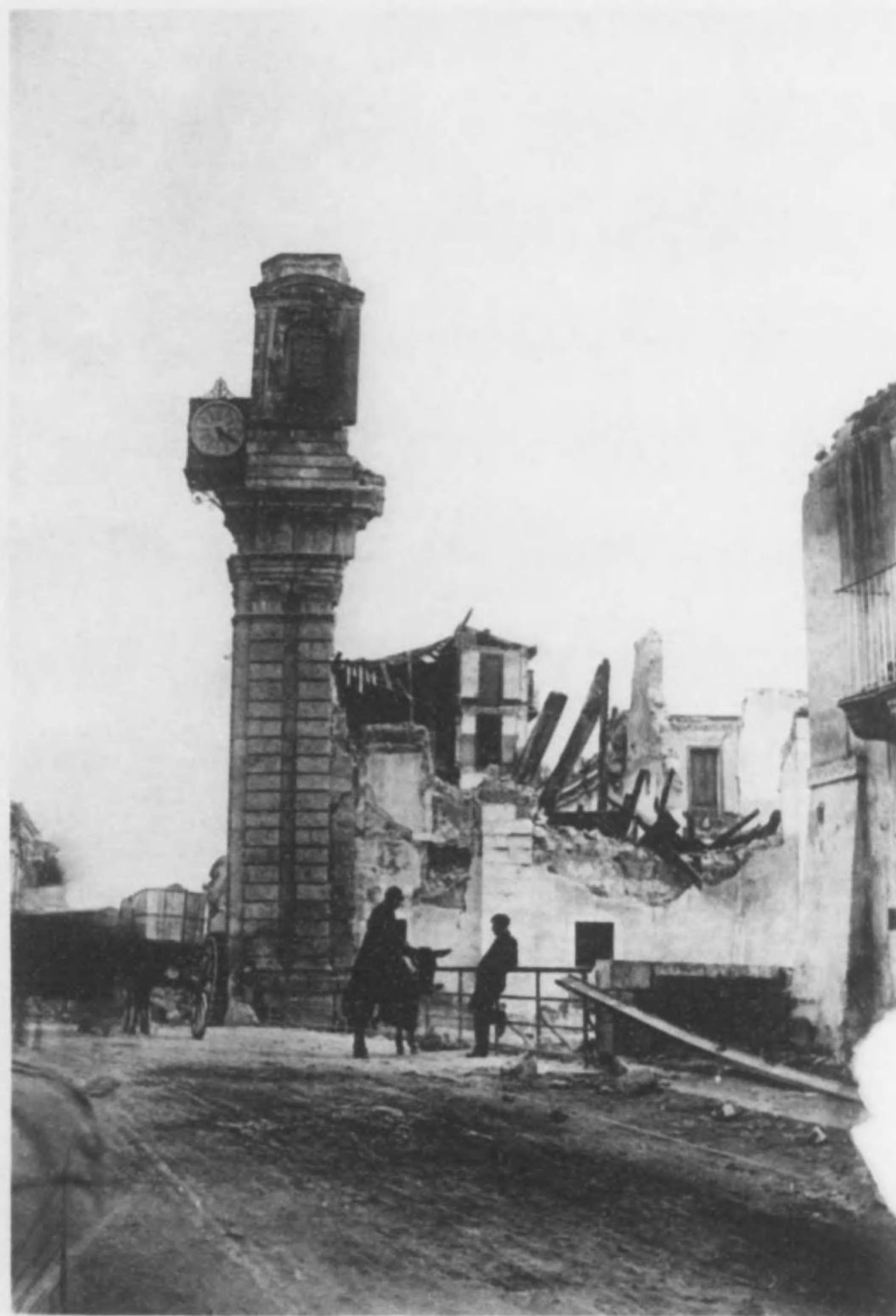
Fig. 6. Messina-Reggio Earthquake of Dec. 28, 1908. A wrecked house on Via Porta Imperiale, Messina. The clock on the corner post indicates the time of earthquake occurrence, 5 h 23 m (morning).
