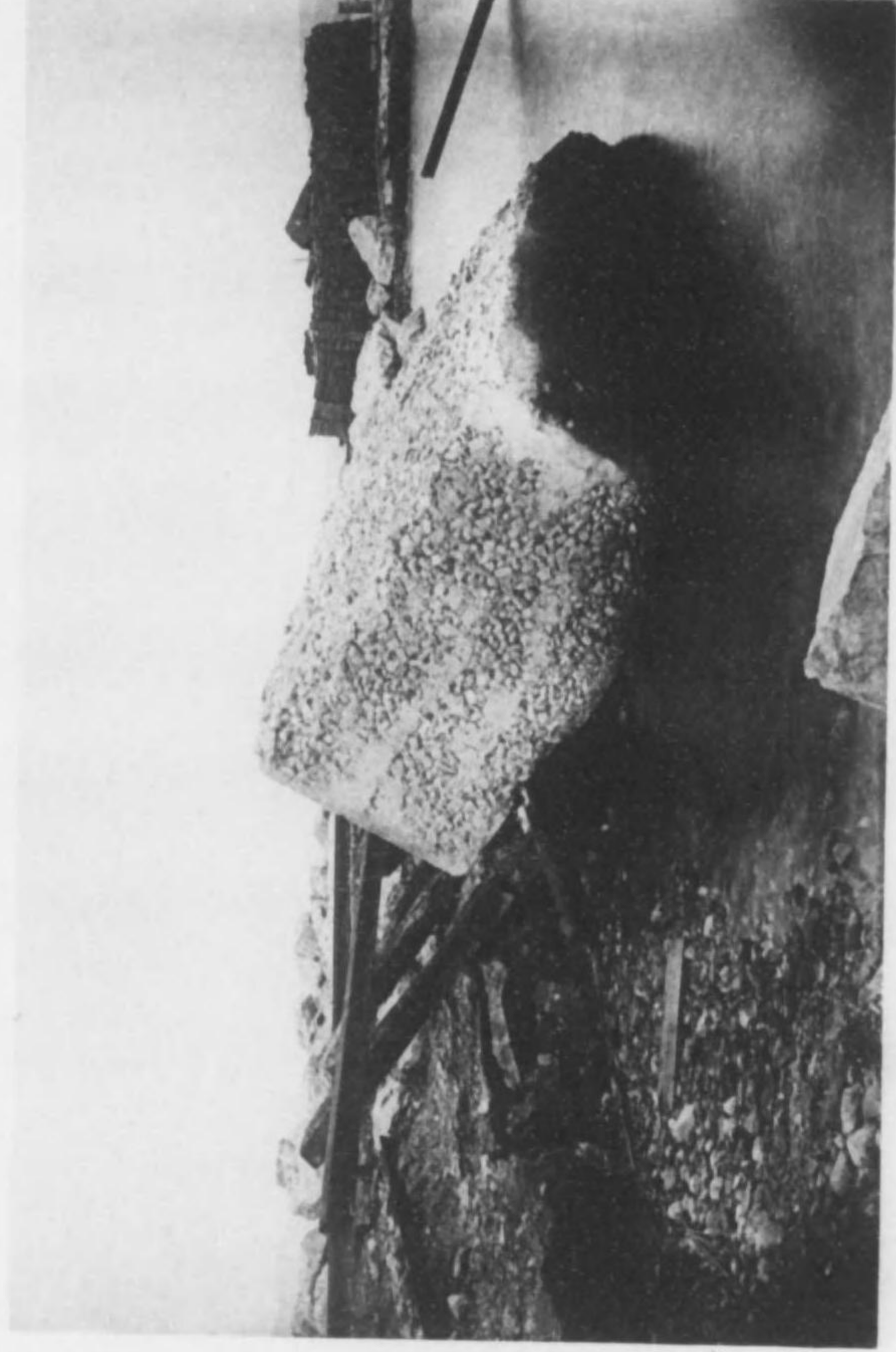
Fig. 9. Messina-Reggio Earthquake of Dec. 28, 1908. Effect of the Isunimi (maremoto), showing a large concrete block (2.6 x 2.5 x 1.2 metres) of of the port of Reggio carried away about 30 metres from its original position.
