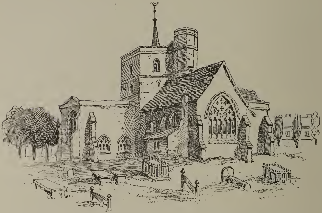
ST. PETER'S CHURCH, BEFORE THE ALTERATIONS OF 1803, FROM THE EAST.
