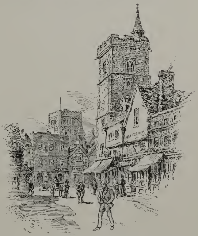
The Clock Tower from the Market Place. From a Drawing by F. G. Kitton.
