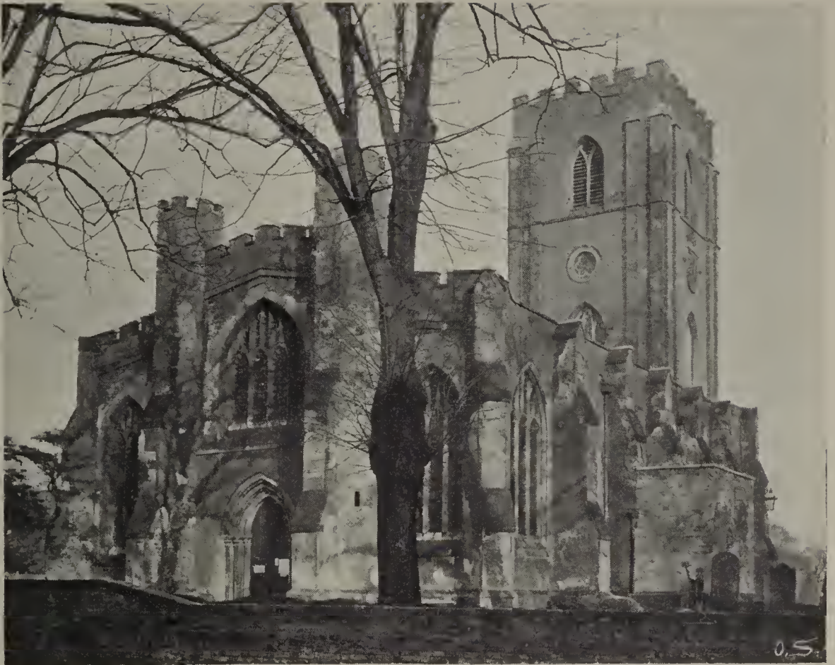
West Front, prior to Lord Grimthorpe's alterations in 1893-94.
