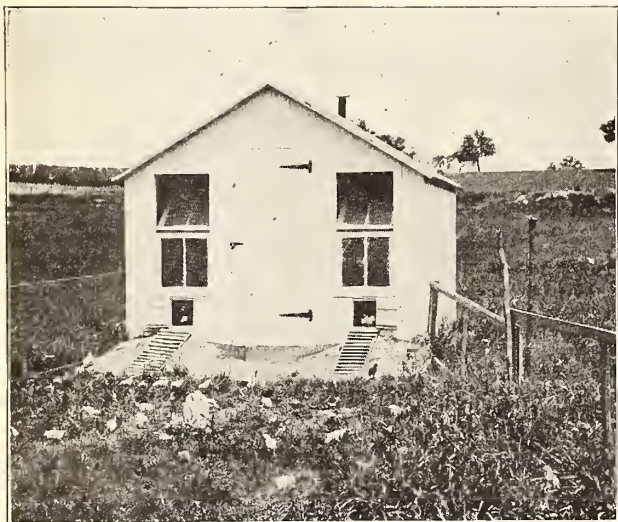
View of colony brooder house using coal-burning brooder stove, U. S. Government poultry farm, Beltsville, Maryland. Yard of portable fencing is shown in front of house. Building instructions may be secured from Poultry Investigations, Bureau of Animal Industry, U. S. Department of Agriculture, Washington, D. C.
