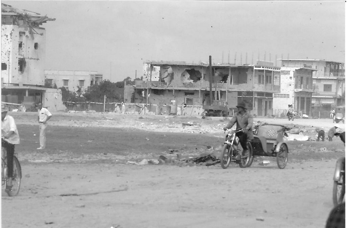
Photo 24 Bomb damage at Can Tho University
